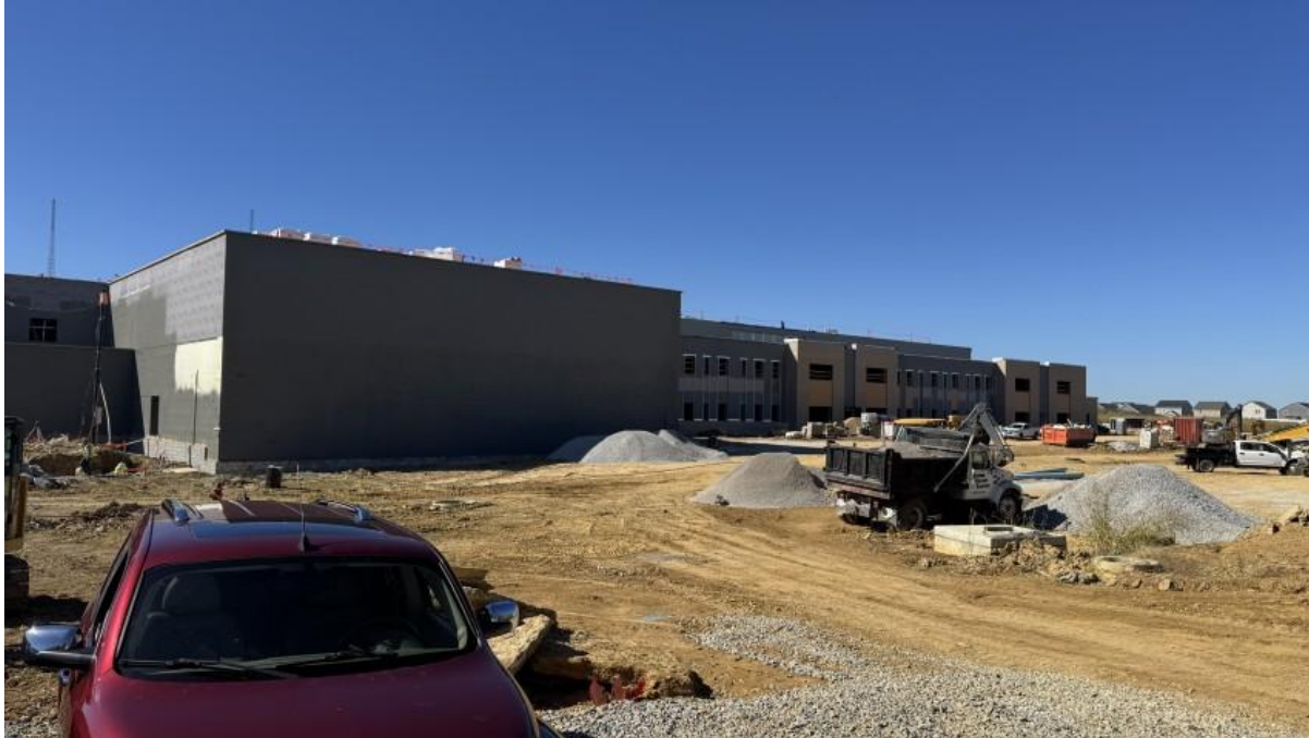
South Face of the Building
