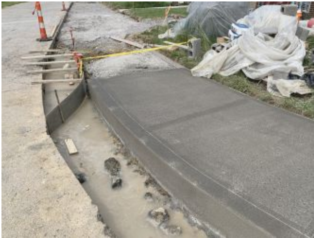
2026.06.25 – New sidewalk looking towards bus loading area
