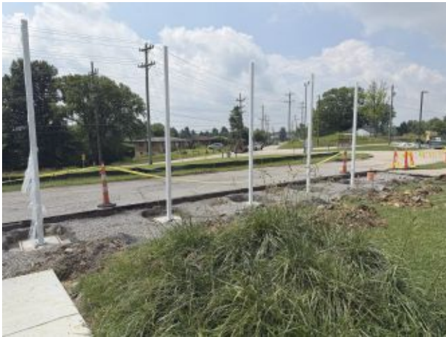
2026.07.09 – Bus canopy posts
