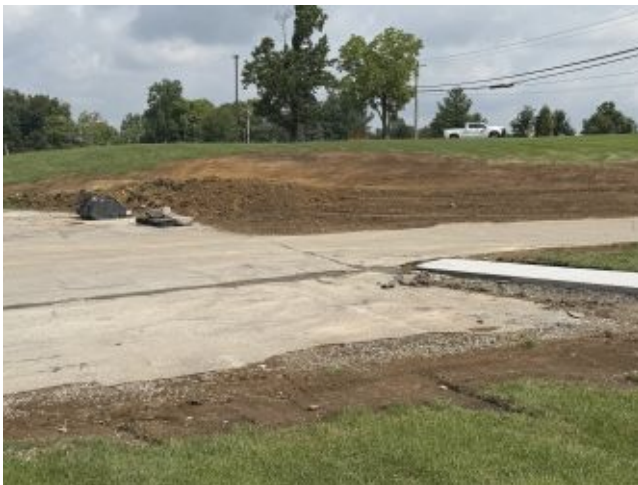
2026.07.09 – North parking lot grading
