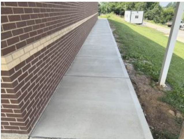
2026.07.09 – New sidewalk north of gym
