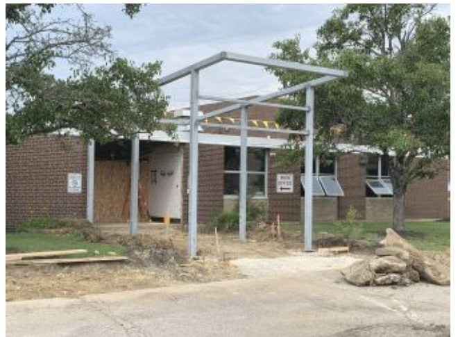
2026.06.25 – New entry canopy structure
