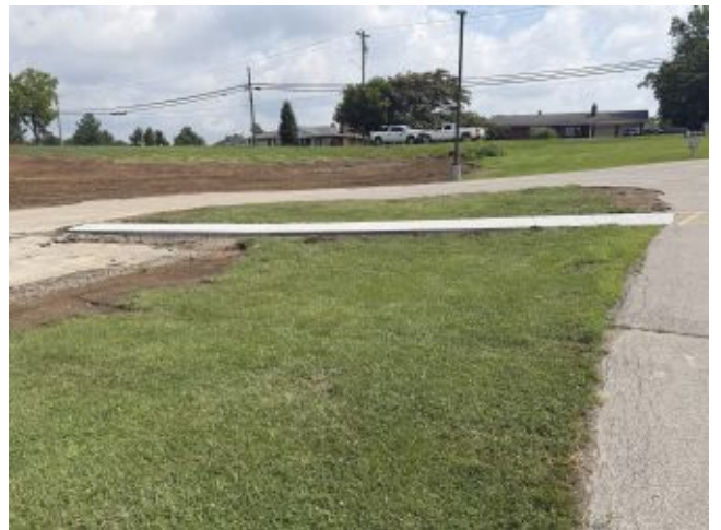
2026.07.09 – New sidewalk at north lot
