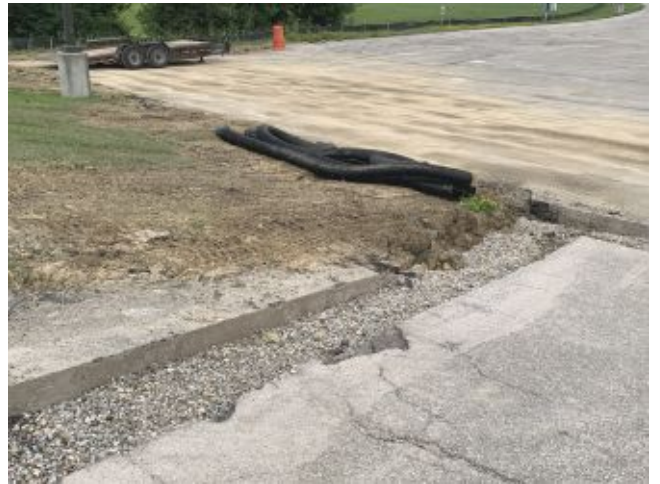
2026.06.25 – Under drain work at north parking lot
