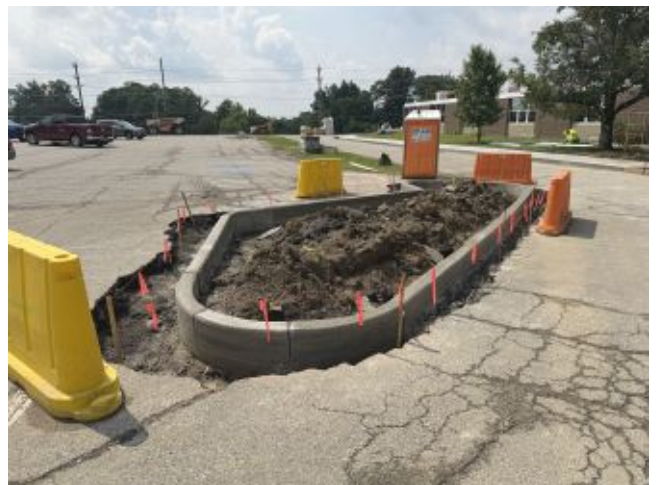
2026.07.09 – Curb near gym entrance
