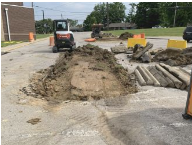
2026.06.25 – Curb demo at main parking lot
