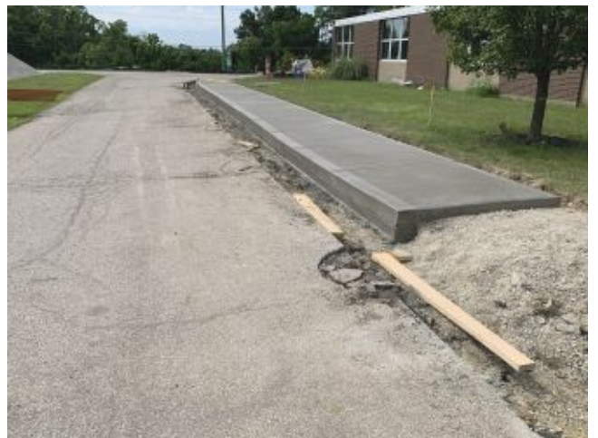
2026.06.25 – New sidewalk south of main entry
