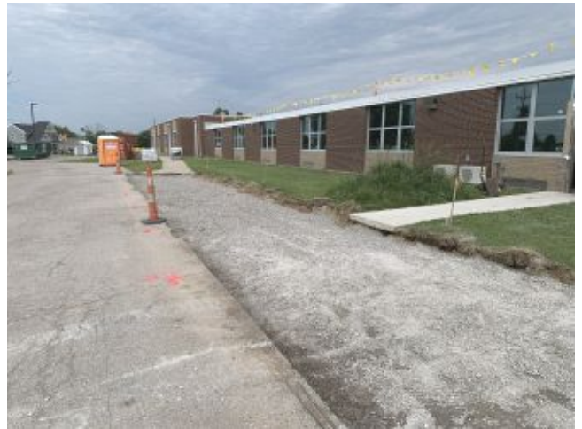
2026.06.25 – Bus loading area
