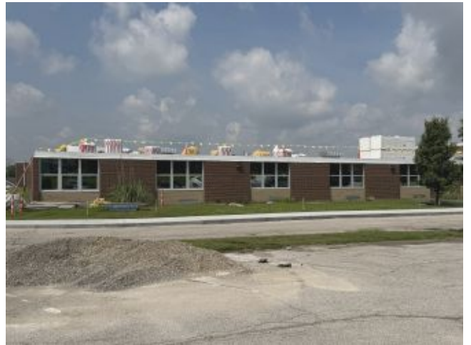
2026.07.09 – Materials staged on roof
