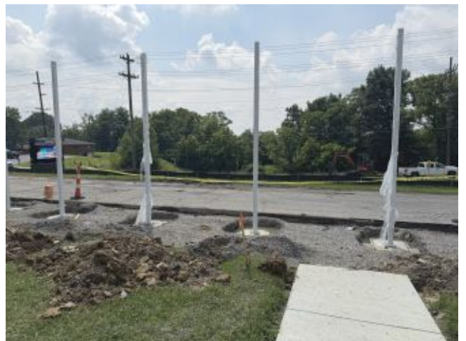
2026.07.09 – Bus canopy posts
