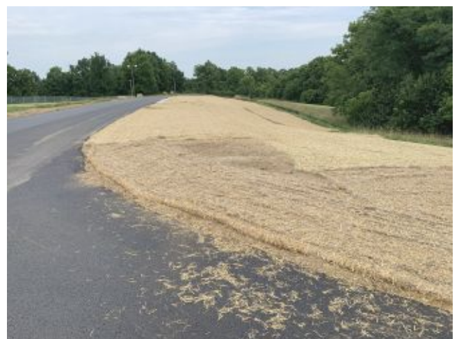
2026.06.25 – Grading at new queue drive
