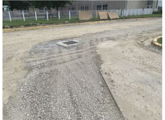
2026.06.30 – Storm laterals in main parking lot
