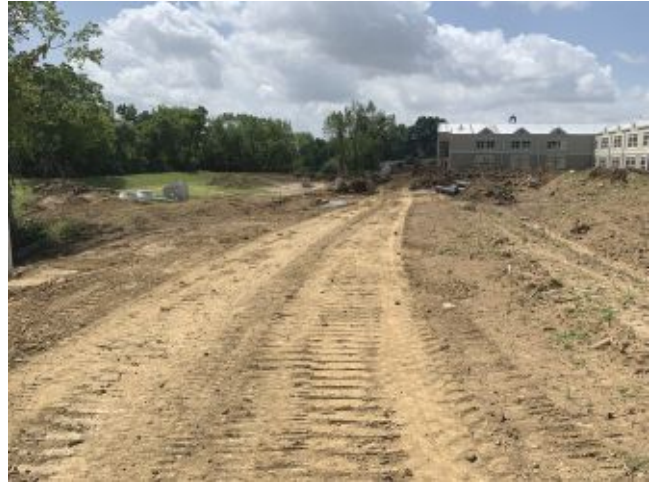
2026.06.30 – East drive from north end of site
