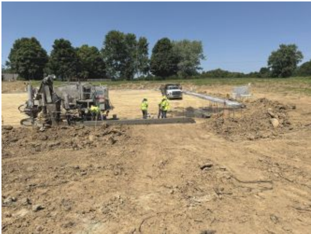
2026.07.14 – Installing curbs at new parking lot
