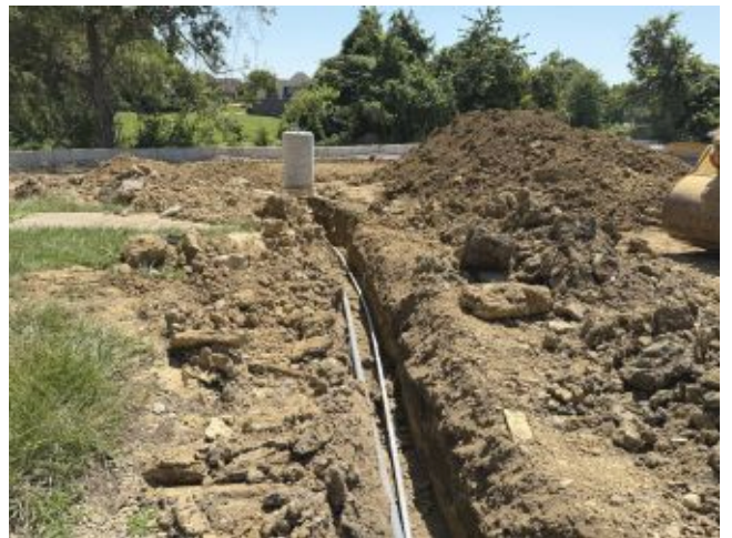
2026.07.14 – Conduit installation at bus loop
