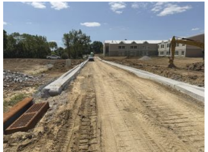
2026.07.23 - East drive from north end of site
