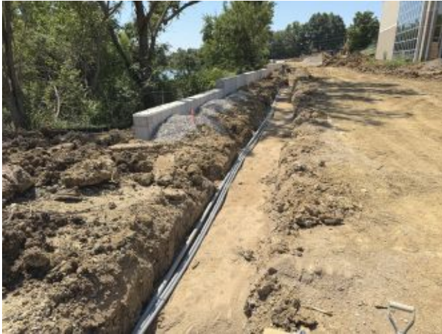
2026.07.14 – Conduits at north end of retaining wall
