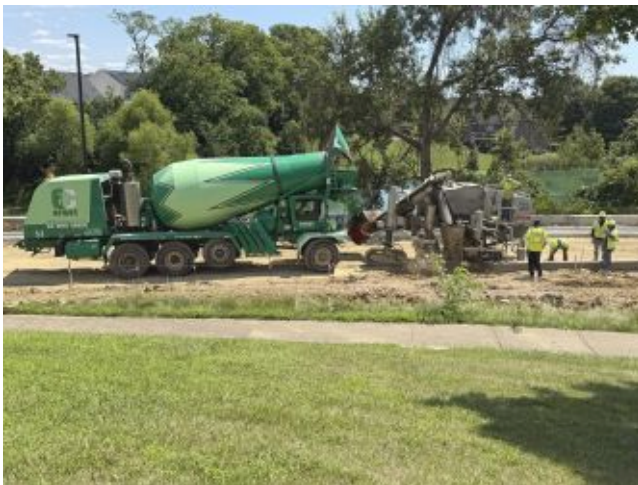
2026.07.23 – Curb crew working on last stretch of curb
