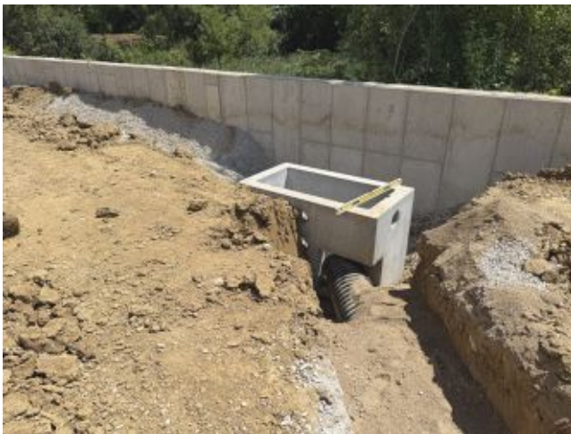
2026.07.14 – Storm structure work east side of site
