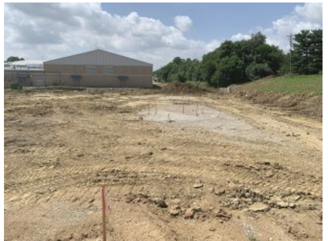
2026.06.30 – West leg of new drive towards new parking lot
