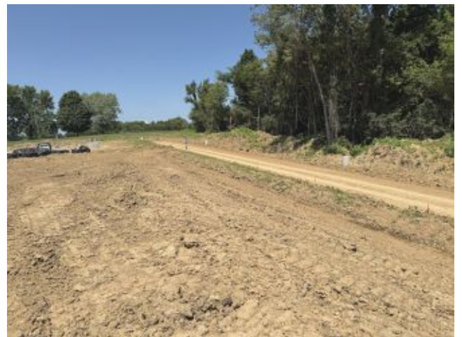
2026.07.14 – North leg of new drive
