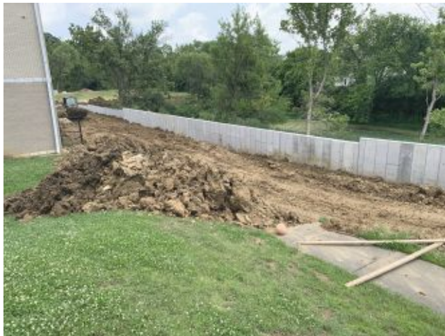
2026.06.30 – New retaining wall
