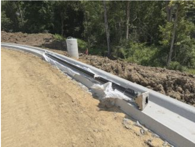
2026.07.23 – Light pole staged for installation
