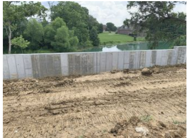
2026.06.30 – New retaining wall
