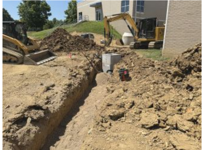
2026.07.14 – Storm structure work east side of site
