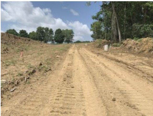
2026.06.30 – North leg of new drive
