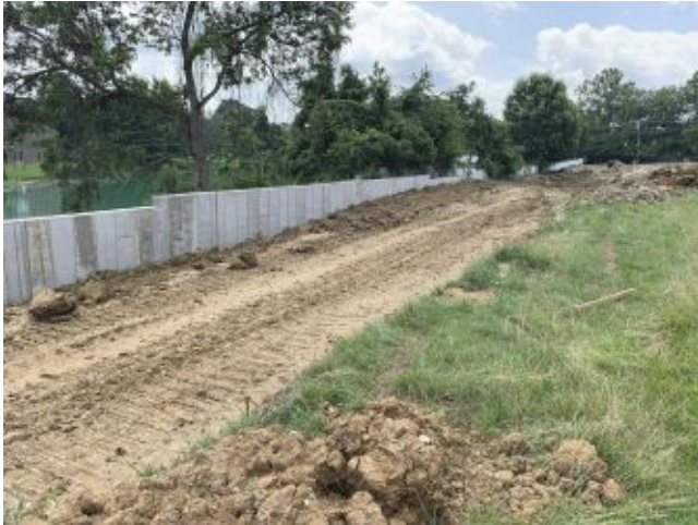
2026.06.30 – New retaining wall
