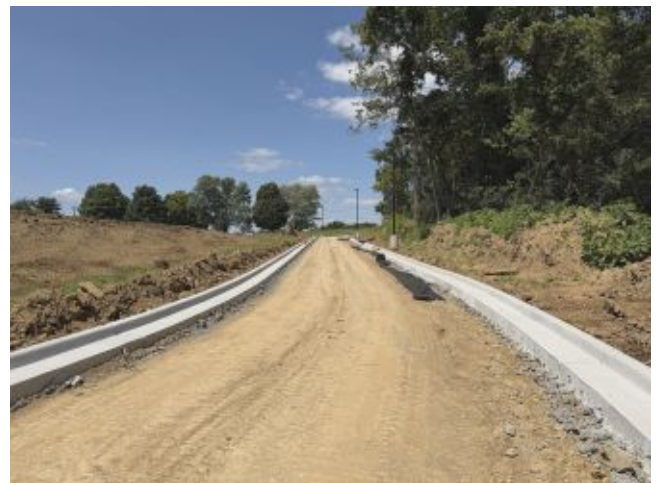
2026.07.23 – North leg of new drive
