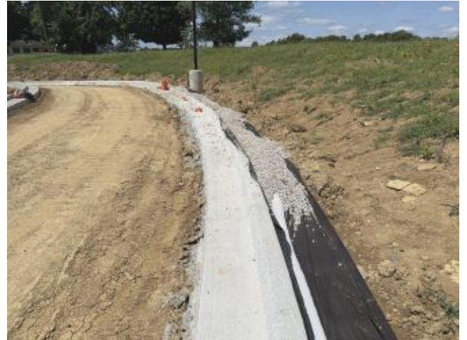
2026.07.23 – Under drain behind curb at northwest corner of site
