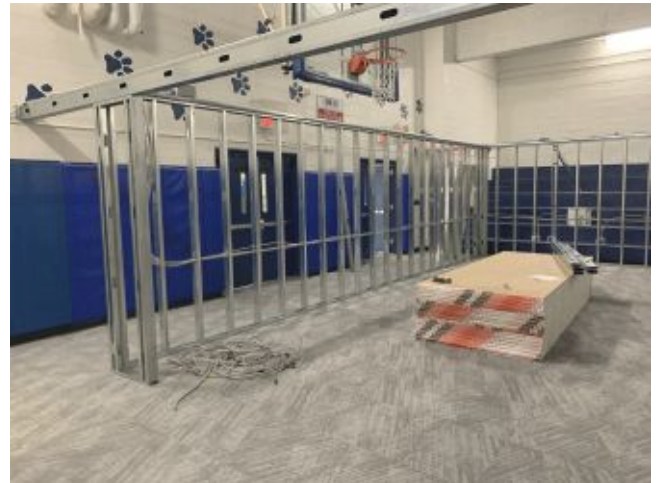
2026.07.02 – Gym temporary classrooms
