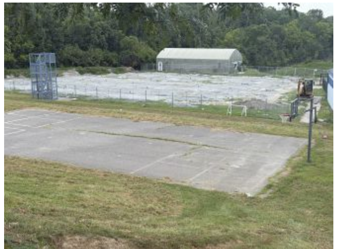
2026.07.16 – Geothermal well field
