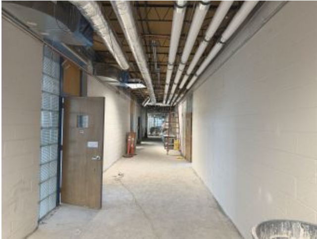
2026.07.16 – Corridor #C200 towards Area C
