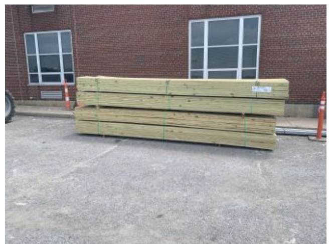
2026.07.02 – Roof blocking staged for installation
