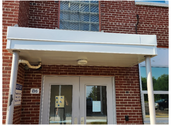
2026.07.17 – New soffit panels, edge flashing, and lighting at exterior canopy.
