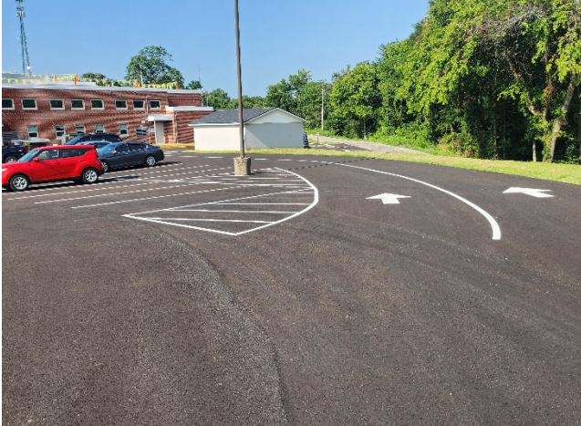
2026.07.17 – Asphalt paving and striping complete.
