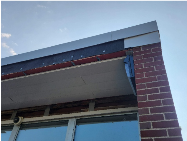
2026.07.17 – Edge flashing being installed at overhang. New soffit panels installed.
