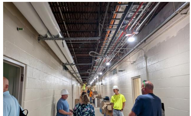
2026.06.23 – Corridor #103 looking west
