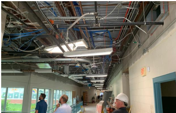
2026.07.07– Corridor #132 looking north
