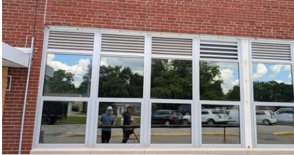
2026.06.23 – New Louver installed in existing Classroom #130 window
