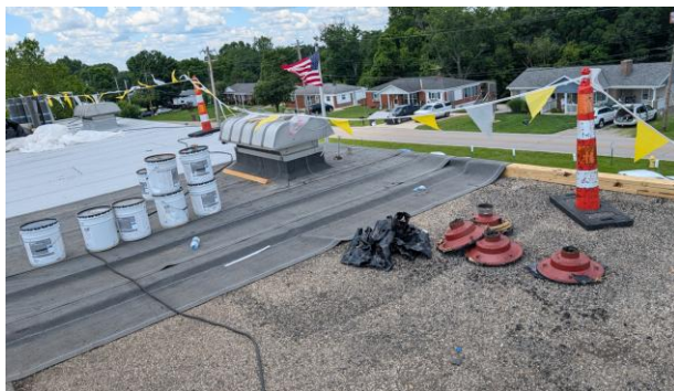
2026.06.23 – New modified bit roofing system and insulation installation above Classrooms
