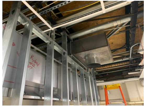
2026.07.07–Kitchen 116 Exhaust Hood Installation
