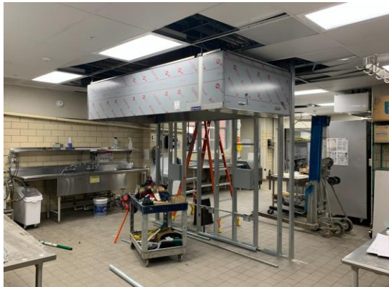
2026.07.07–Kitchen 116 Exhaust Hood Installation
