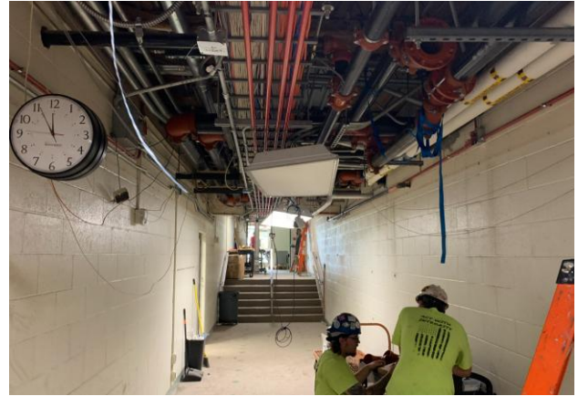
2026.07.07– Corridor #104 looking north
