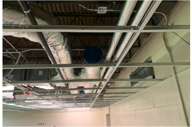
2026.07.07 – Classroom #127 Ceiling Grid Install
