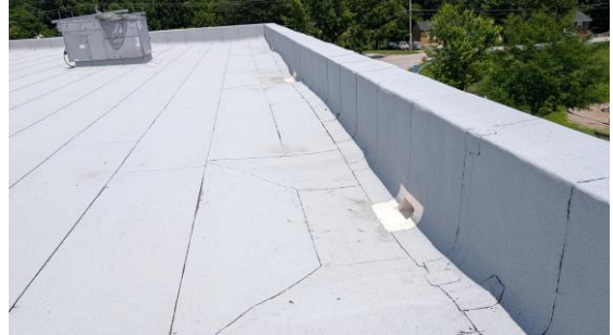
2026.06.23 – New modified bit roofing system and insulation installed above Gym
