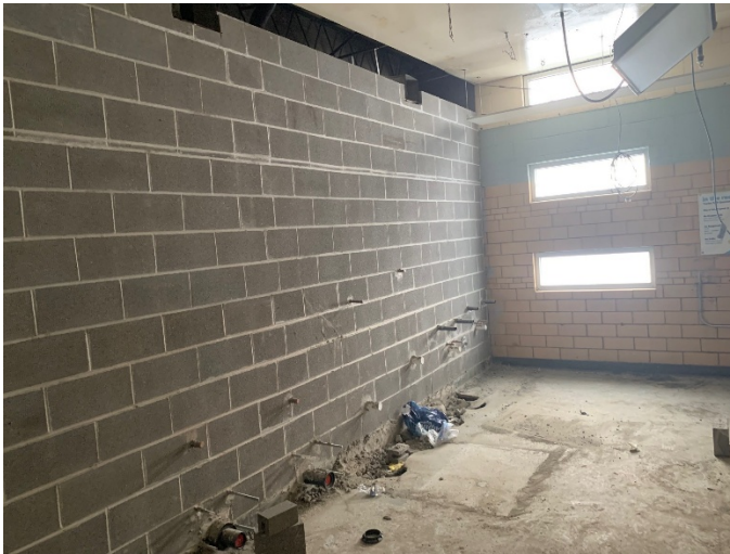
2026.07.08 – Front wing boys restroom – new cmu wall
