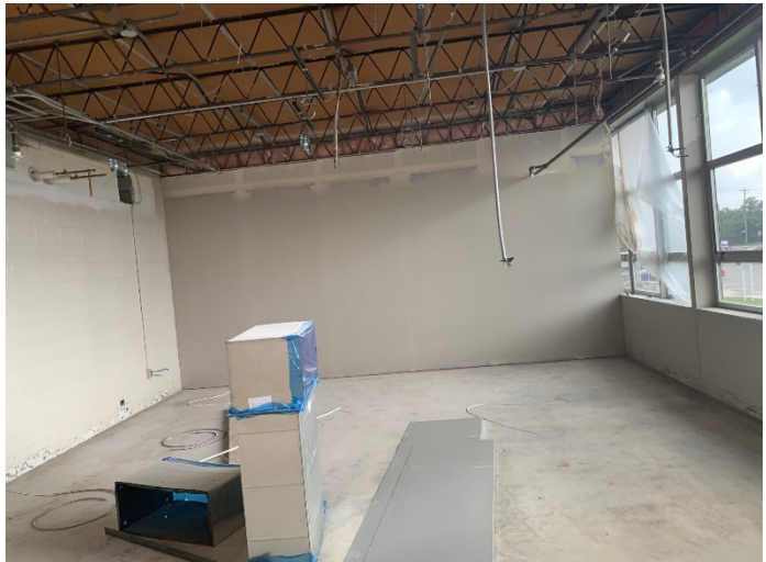
2026.07.08 – Front wing typical classroom-street side
