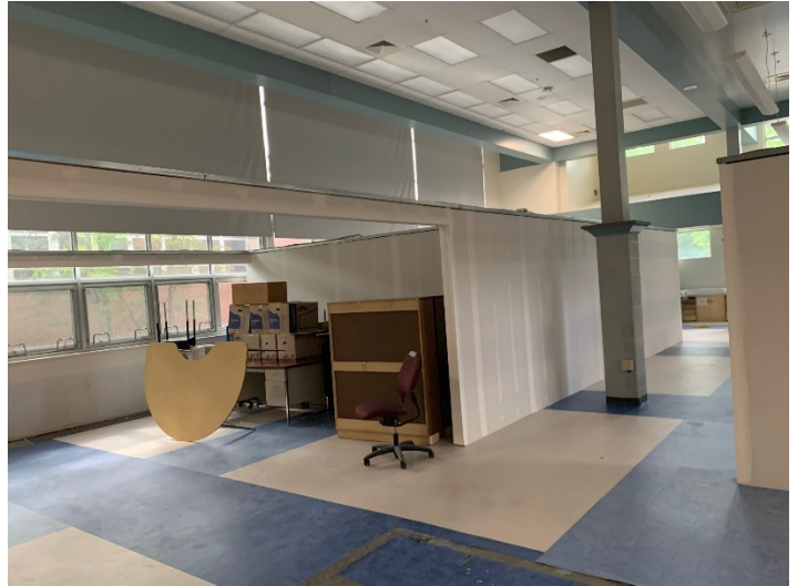
2026.07.08 – Temporary classrooms – media center
