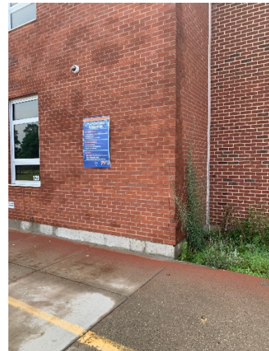
2026.07.08 – Brick cleaning – rear wing
