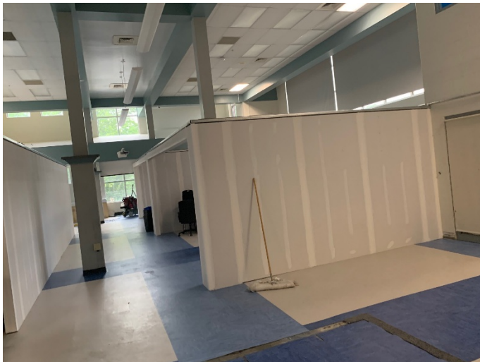
2026.07.08 – Temporary classrooms – media center
