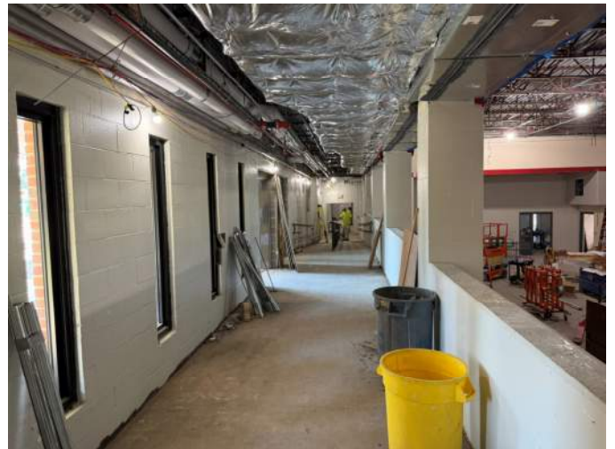
2026.07.14 – Phase 4 corridor along cafeteria
