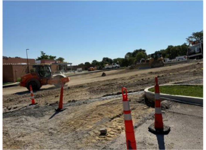
2026.07.14 – South parking lot paving removal
