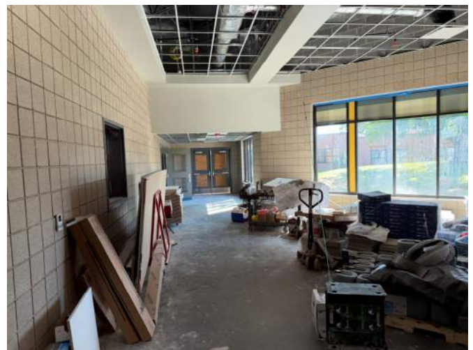
2026.07.14 – New addition main corridor/flex area
