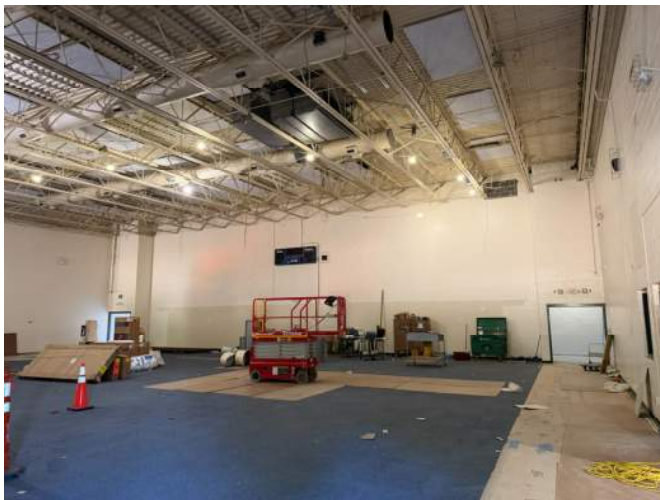
2026.07.14 – Gym – acoustic panel installation on roof deck
