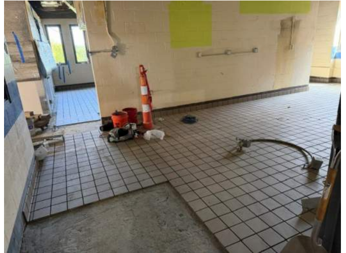
2026.07.14 – Kitchen – new quarry tile floor
