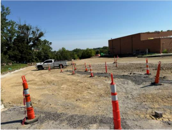
2026.07.14 – West parking lot paving removal
