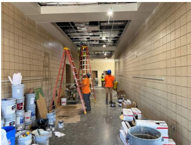
2026.07.14 – New addition main corridor
