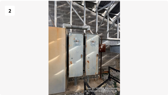
Contactor Cabinets
