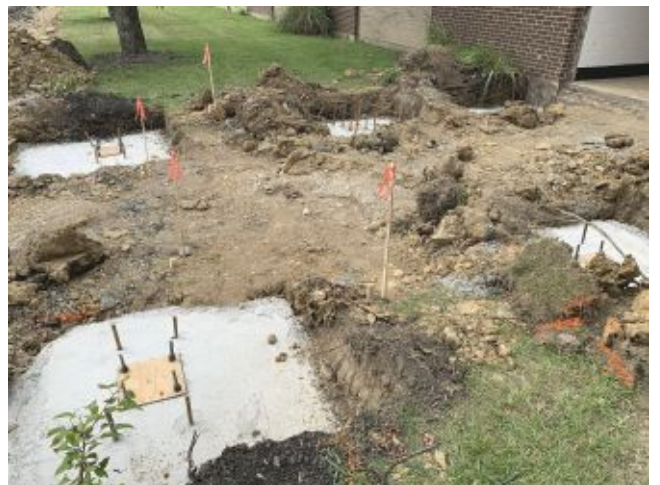
2026.06.11 – New canopy footings
