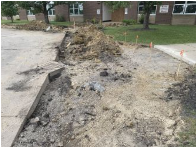
2026.06.11 – Gym entrance sidewalk demo
