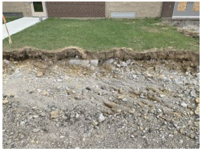
2026.06.11 – Bus canopy sidewalk demo
