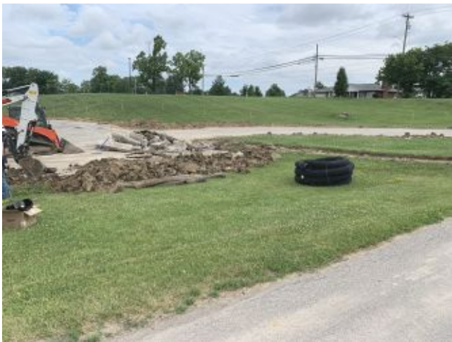
2026.06.11 – Parking lot curb demo
