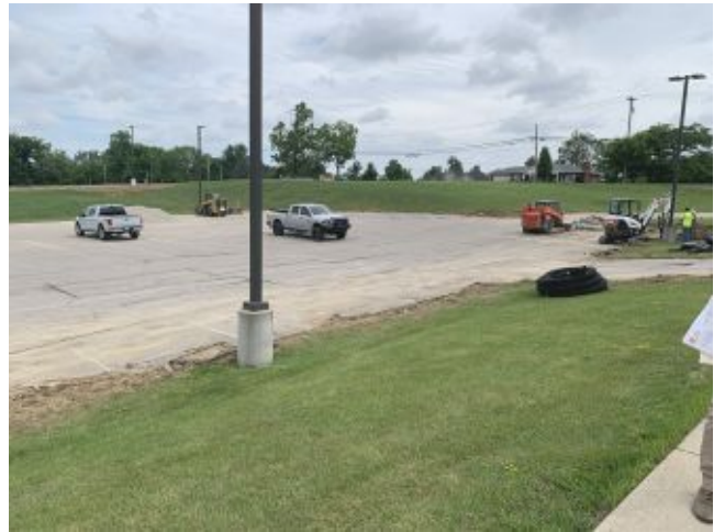
2026.06.11 – Parking lot curb demo
