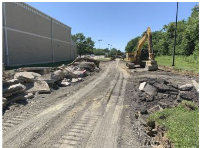
2026.06.02 – Demolished curbs along west side of gymnasium
