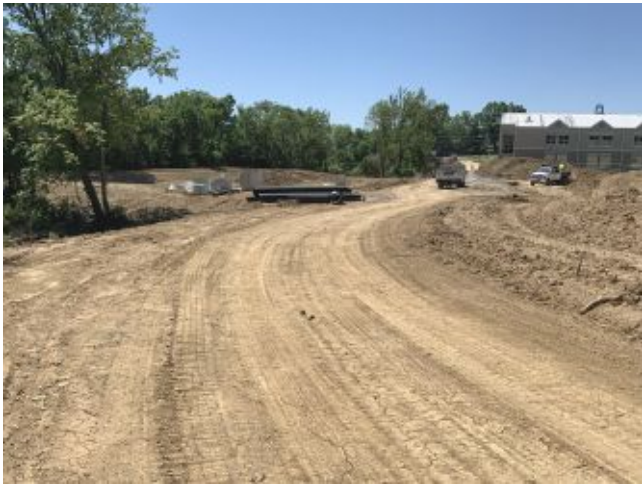
2026.06.02 – East drive from north end of site
