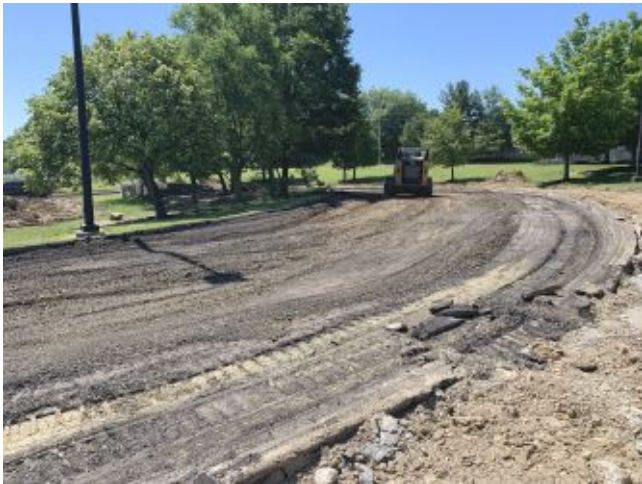
2026.06.02 – Bus loop demolition
