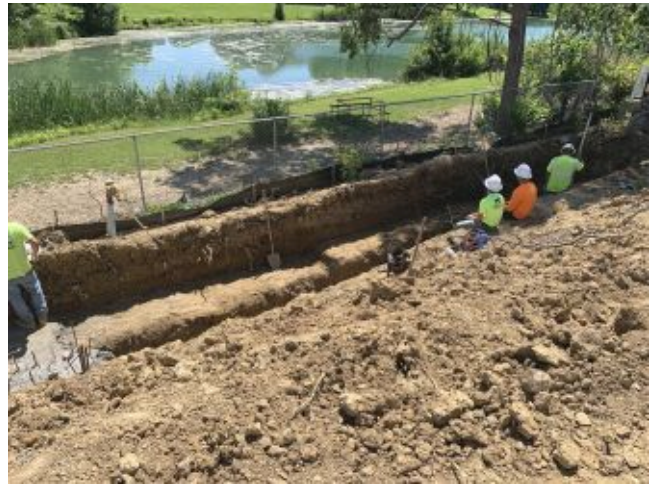
2026.06.02 – Retaining wall footing
