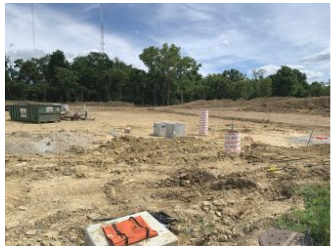
2026.06.16 – New parking lot
