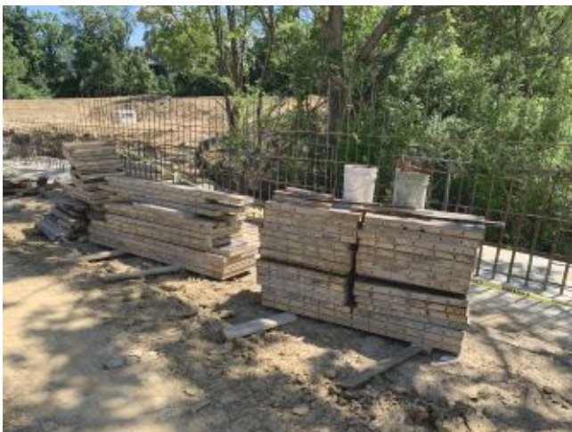
2026.06.02 – Retaining wall forms
