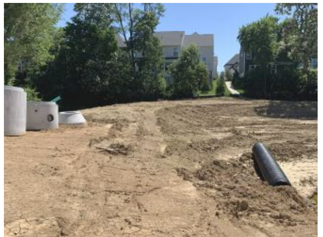
2026.06.02 – North end of detention pond
