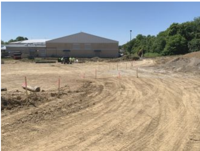
2026.06.02 – West leg of new drive towards new parking lot
