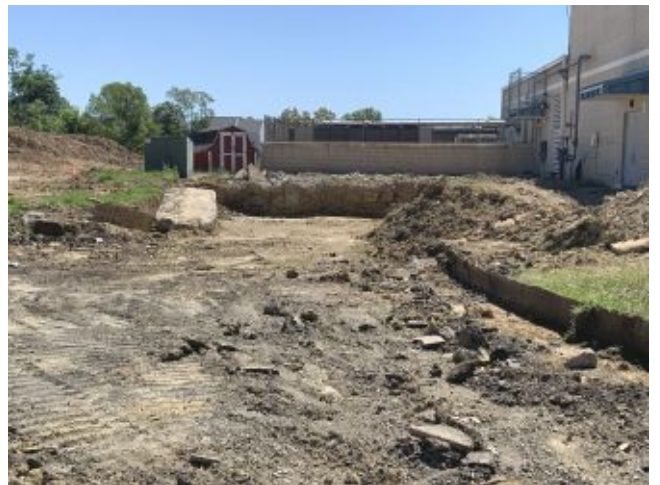
2026.06.02 – Loading dock demolition
