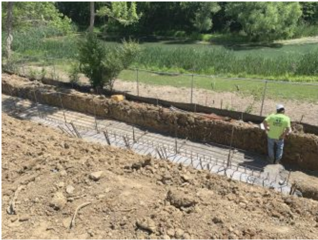
2026.06.02 – Retaining wall footing
