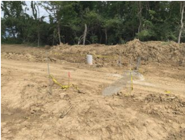
2026.06.16 – Light pole base north leg of drive
