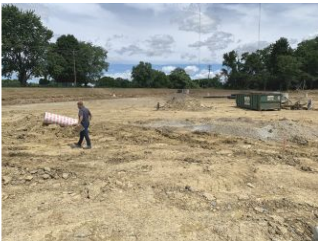
2026.06.16 – New parking lot
