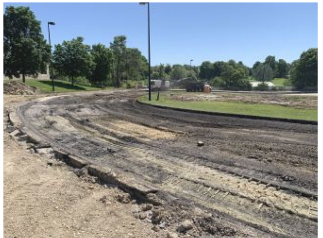
2026.06.02 – Bus loop demolition
