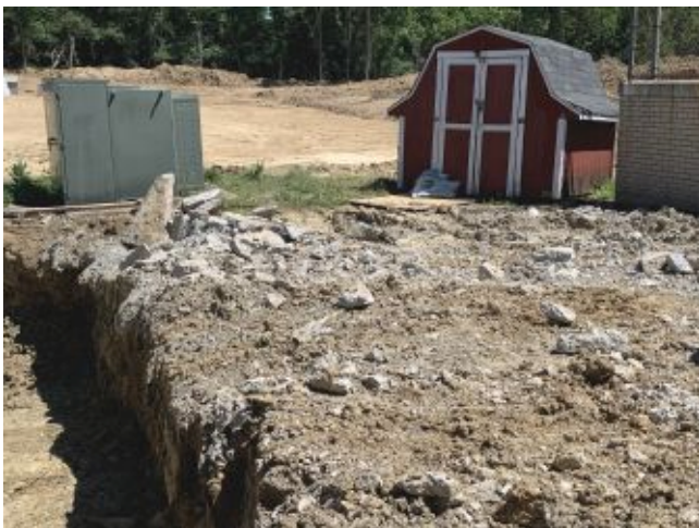
2026.06.02 – Loading dock demolition
