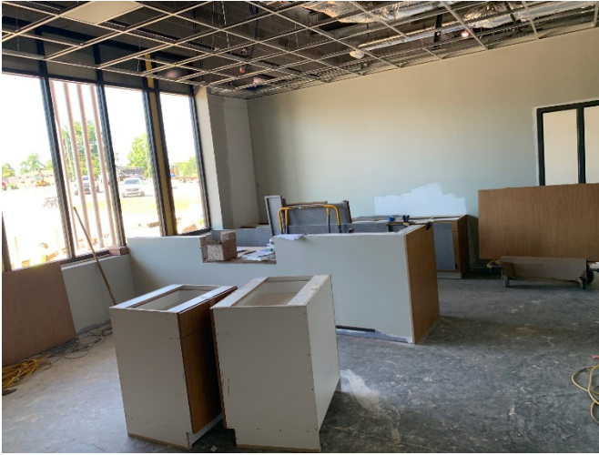
2026.06.16 – New addition-Reception area
