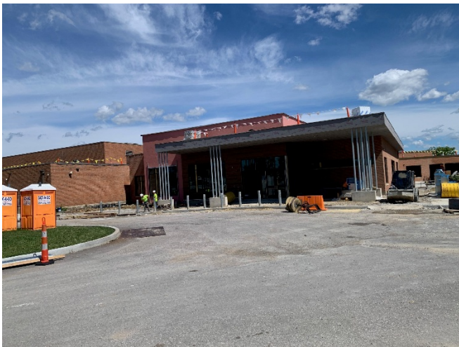
2026.06.16 – New addition – bollard install
