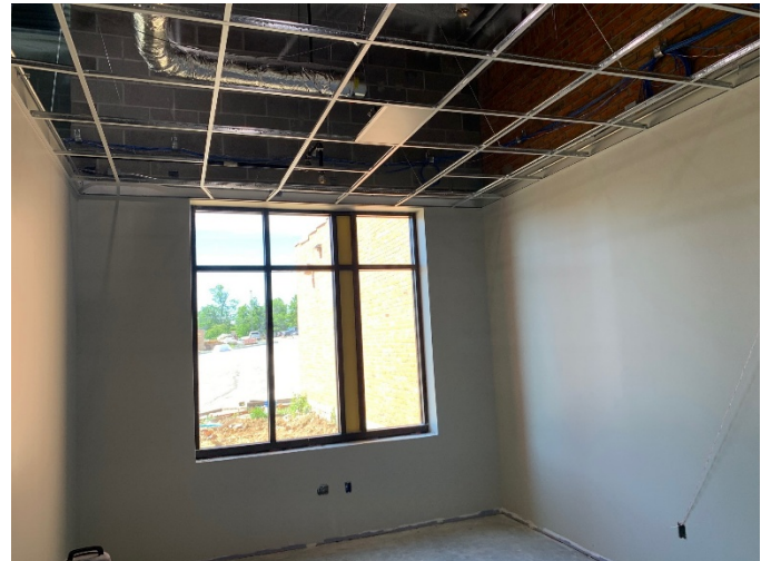
2026.06.16 – New addition-conference room
