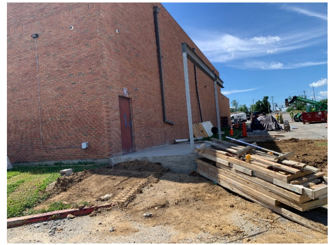
2026.06.16 – Gym vestibule structural steel/foundation
