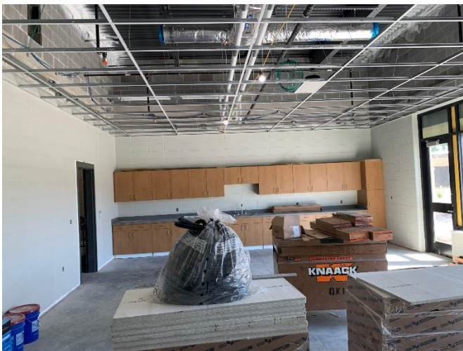
2026.06.16 – New addition-Art classroom
