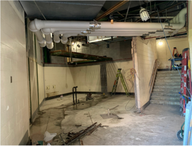
2026.06.16 – Cafeteria bathrooms demolition
