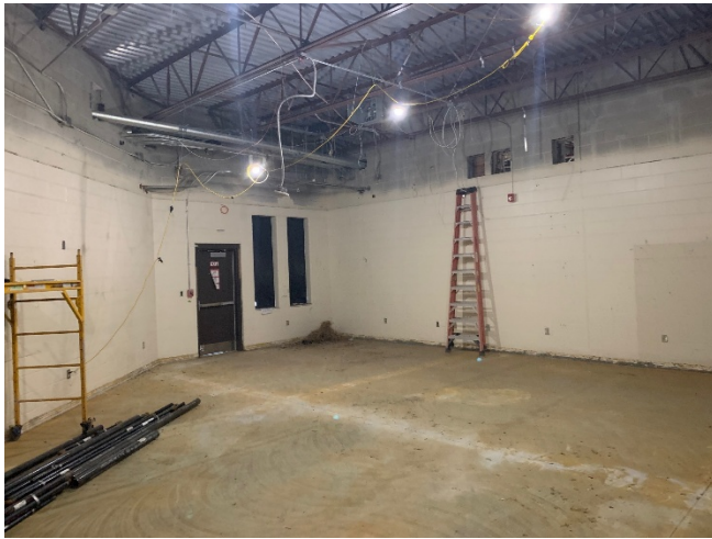
2026.06.02 – Music room demolition
