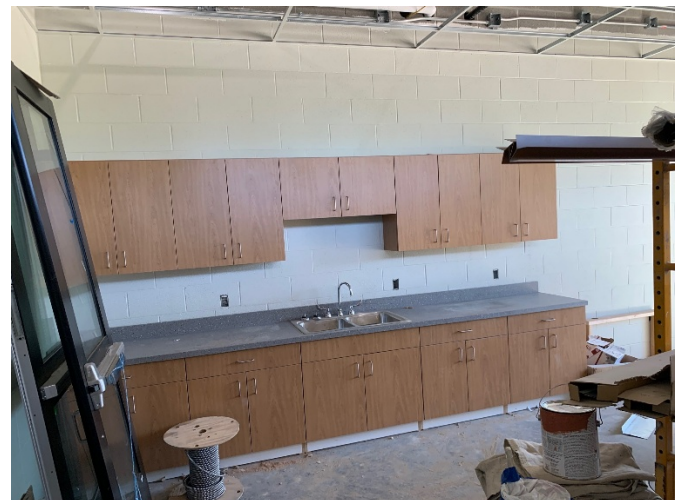
2026.06.16 – New addition-staff workroom
