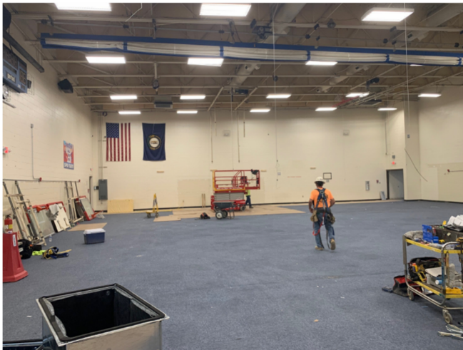
2026.06 02 – Gym equipment demolition
