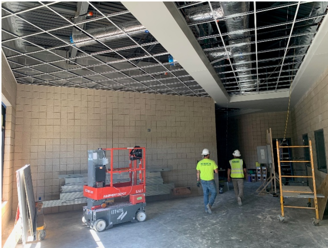
2026.06.02 – New addition-Flex area
