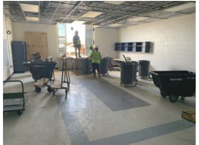
2026.06.04 – Debris removal Classroom #214
