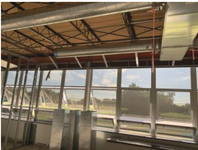
2026.06.16 – Ductwork installation in Classroom #201
