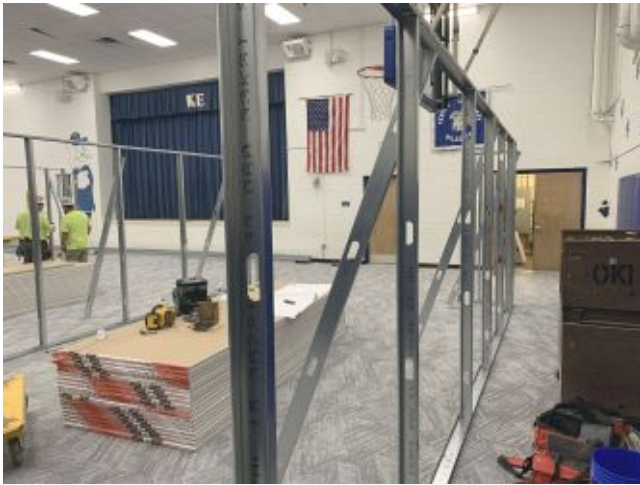
2026.06.18 – Gym temporary classroom framing
