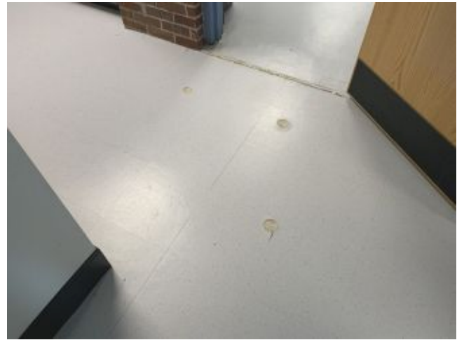
2026.06.18 – General office slab jacking locations
