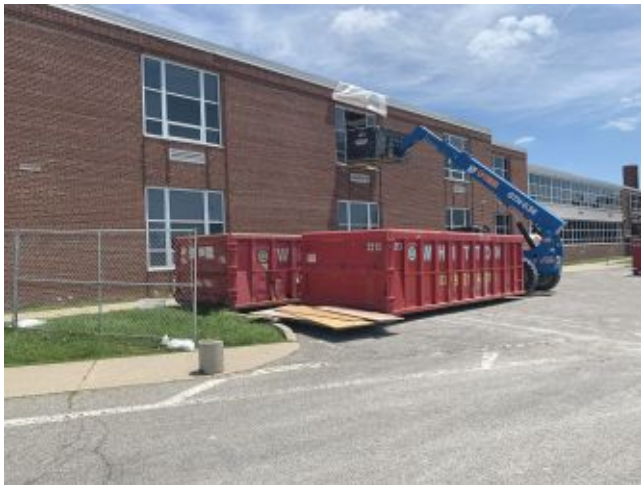
2026.06.04 – Debris removal from 2 nd floor
