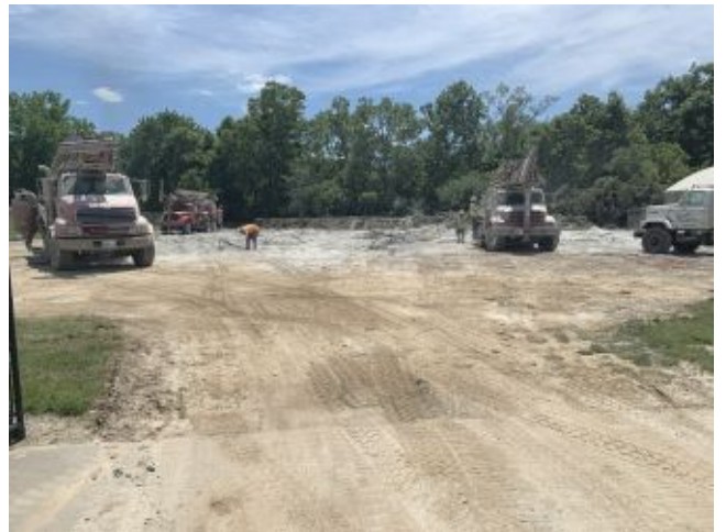
2026.06.04 – Geothermal well field installation
