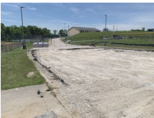
2026.06.04 – Removed asphalt parking
