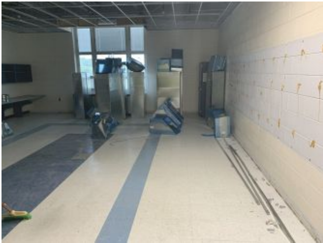
2026.06.04 – Ductwork staged in Classroom #212
