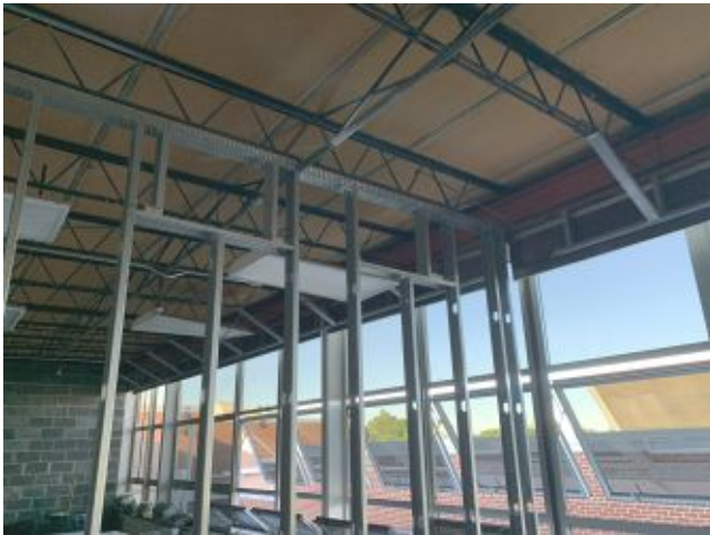
2026.06.16 – Framing between Classrooms #204 & #206
