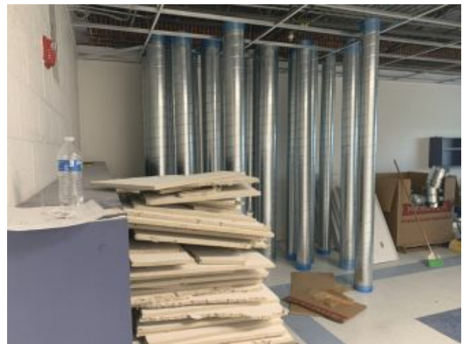
2026.06.04 – Ductwork staged in Classroom #212
