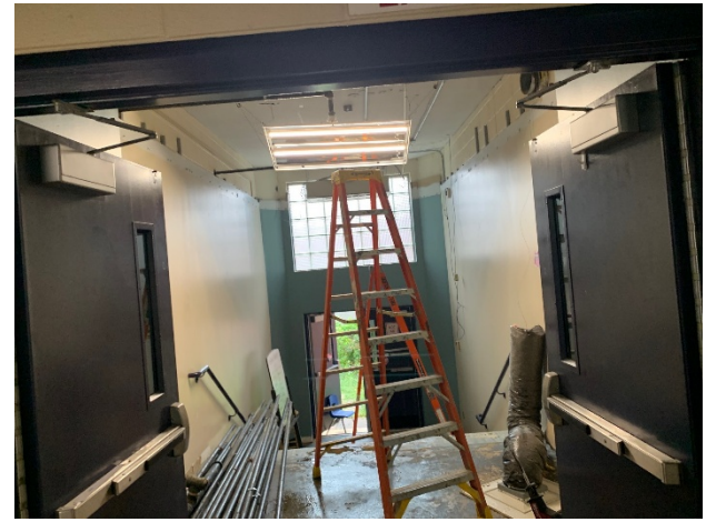
2026.06.09 – Stair to courtyard demolition
