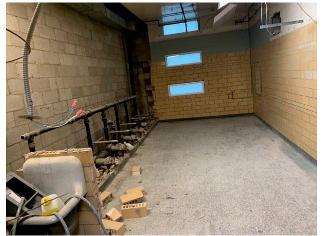
2026.06.09 – Girls restroom demolition
