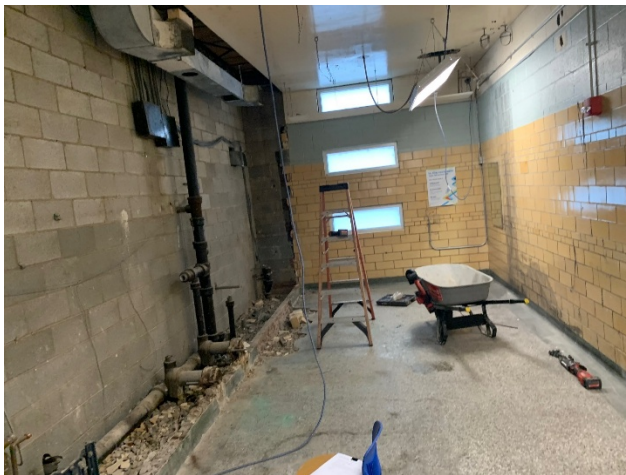
2026.06.09 – Boys restroom demolition
