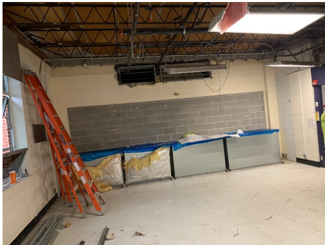
2026.06.09 – Art classroom demolition
