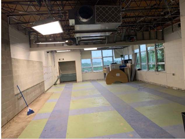
2026.06.09 – Phase 1B-front preschool room demolition
