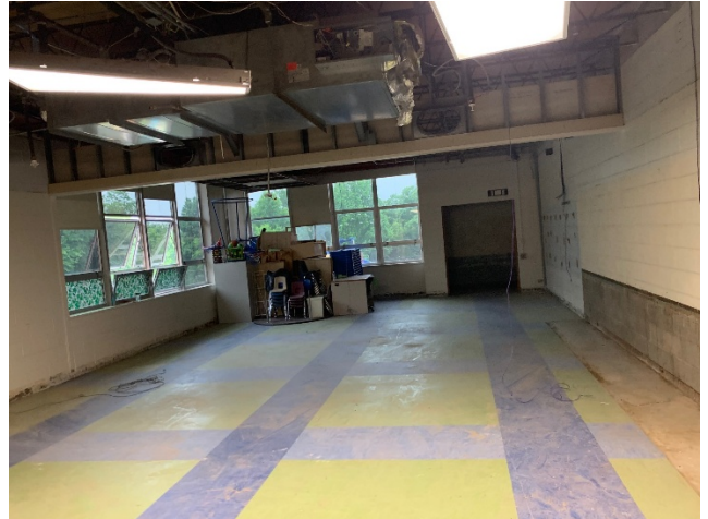
2026.06.09 – Phase 1B-rear preschool room demolition
