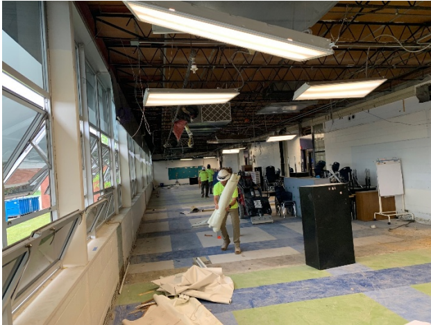
2026.06.09 – Phase 1A/1B front classrooms wing demolition (front)
