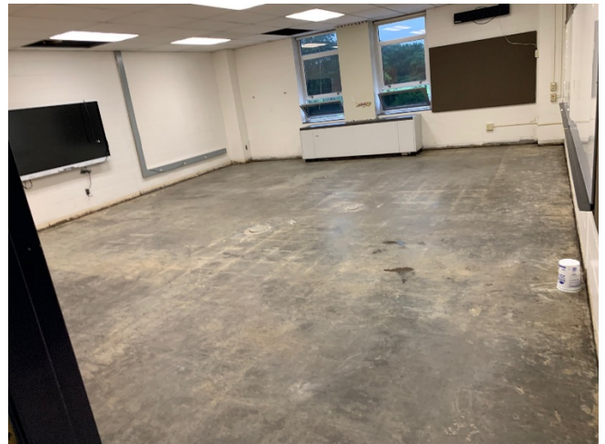
2026.06.09 – Rear wing classroom - floor tile asbestos abatement
