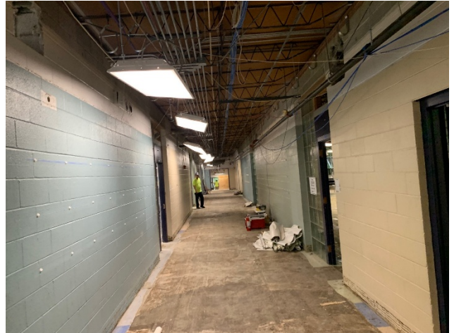
2026.06.09 – Phase 1A/1B front corridor demolition
