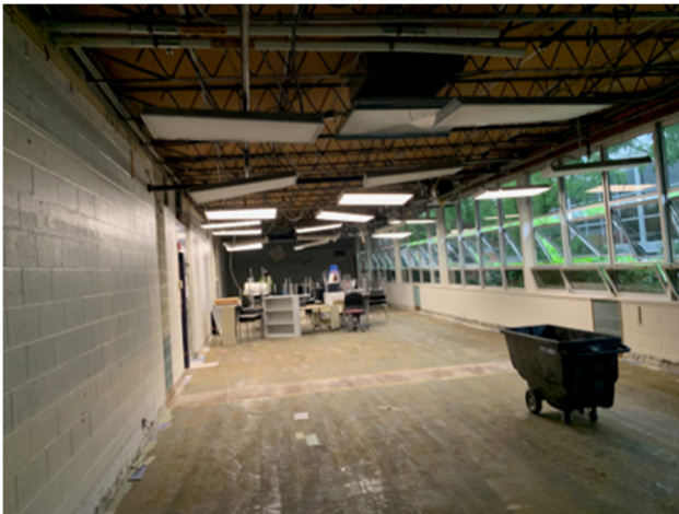
2026.06.09 – Phase 1A/1B front classroom wing (rear) demolition
