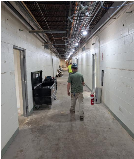
2026.06.09 – Corridor #103 looking west
