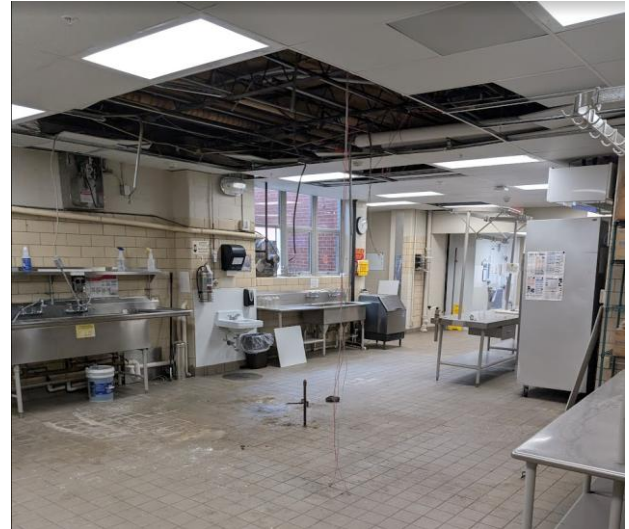
2026.06.09–Kitchen 116 Exhaust Hood Removed
