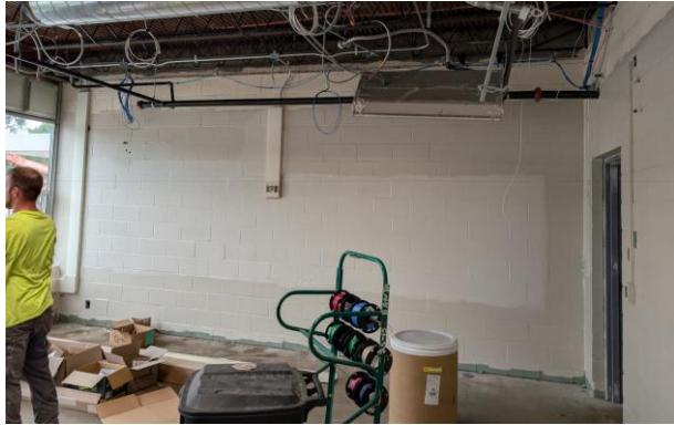
2026.06.09– Classroom #130 looking east
