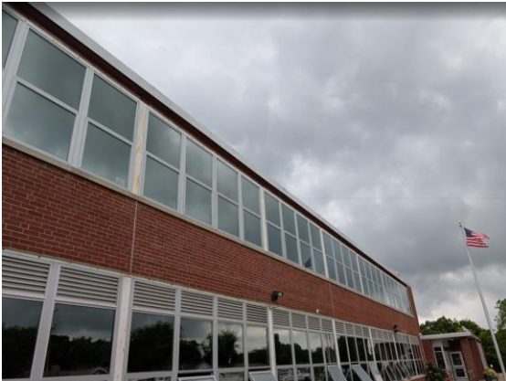
2026.06.09 – Transite panels removed above windows
