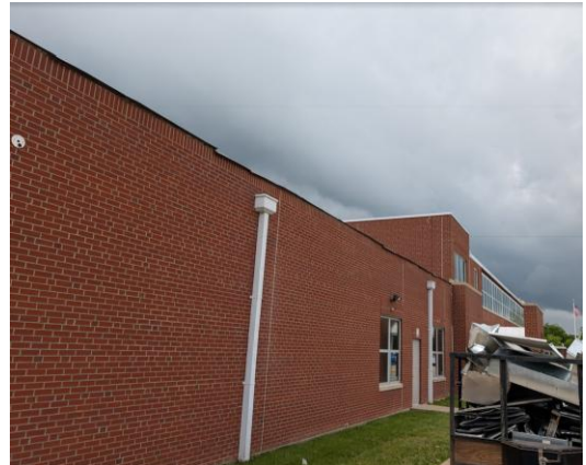
2026.06.09 – Copings removed from parapet
