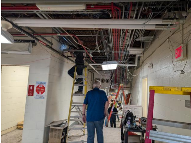
2026.06.09– Corridor #104 looking south
