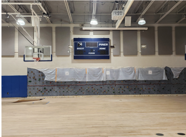
2026.06.09 – Wall acoustic panels, scoreboard, projector screen installed.
