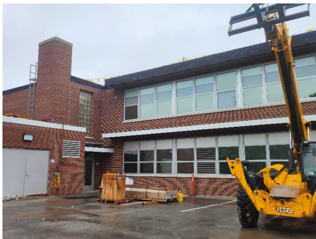
2026.06.09 – Roof work underway on main roof
