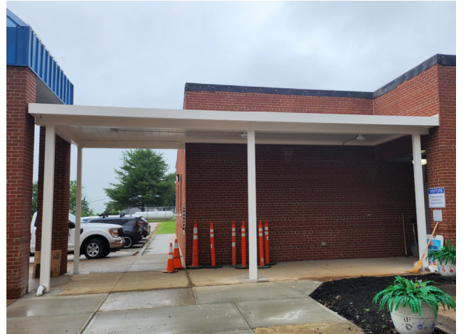
2026.06.09 – New exterior canopy at library entrance.
