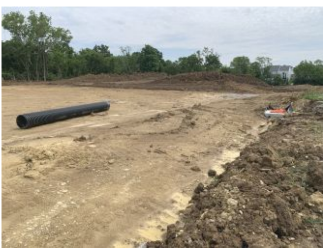
2026.05.19 – New parking lot
