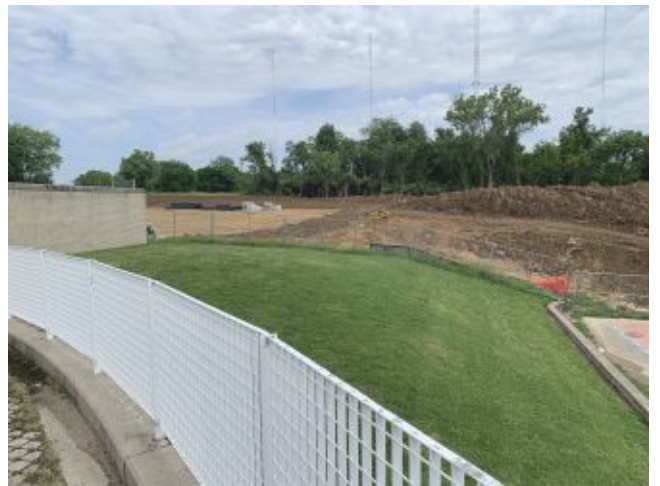
2026.05.19 – Looking northwest from cafeteria
