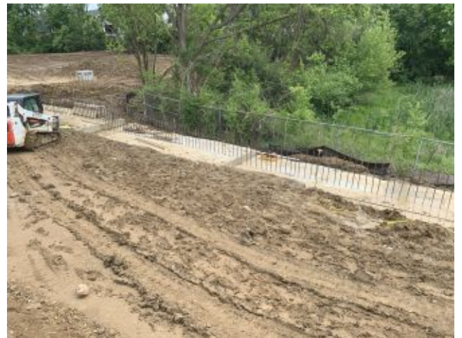
2026.05.19 – Retaining wall footing
