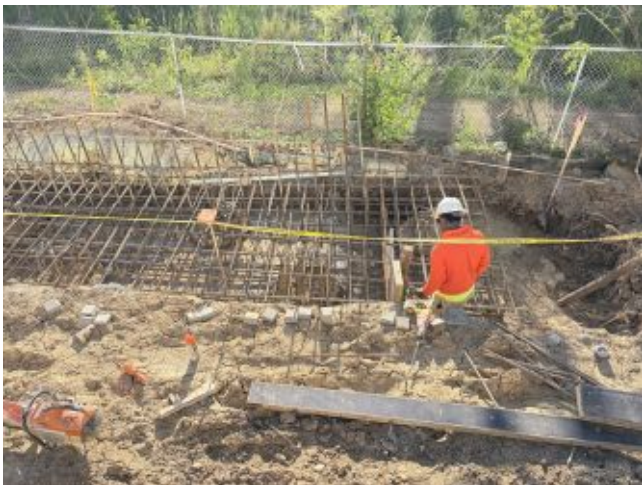
2026.05.07 – Retaining wall footing
