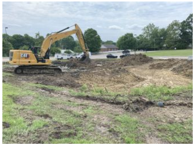
2026.05.19 – Earthwork at bus loop basin
