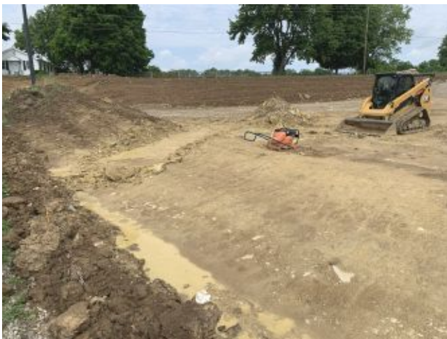
2026.05.19 – New parking lot
