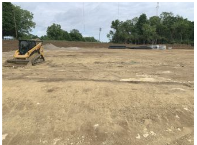
2026.05.19 – New parking lot
