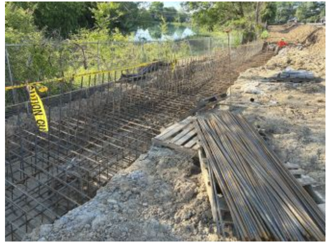
2026.05.07 – Retaining wall footing
