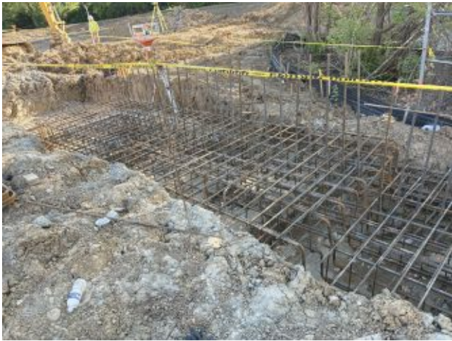
2026.05.07 – Retaining wall footing
