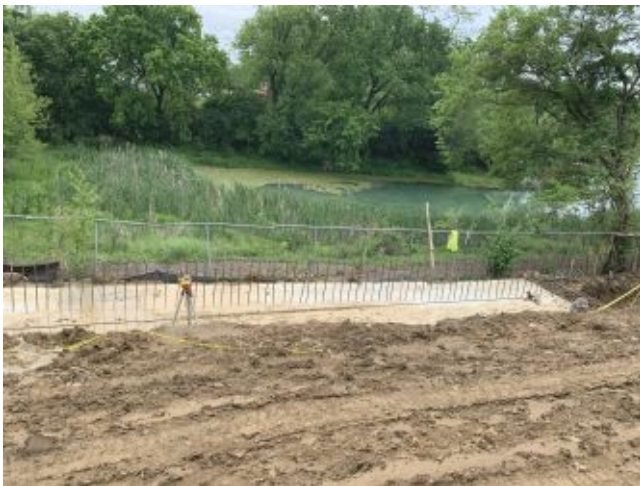
2026.05.19 – Retaining wall footing
