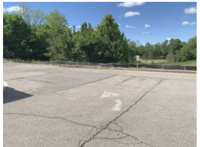
2026.05.04 – Erosion control measures
