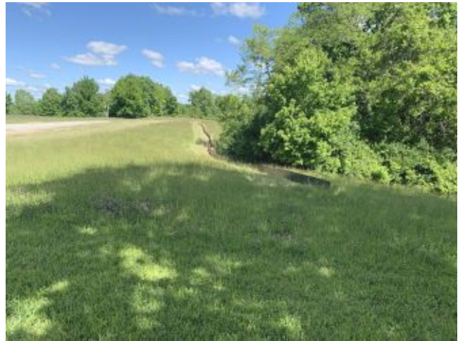
2026.05.04 – Erosion control measures
