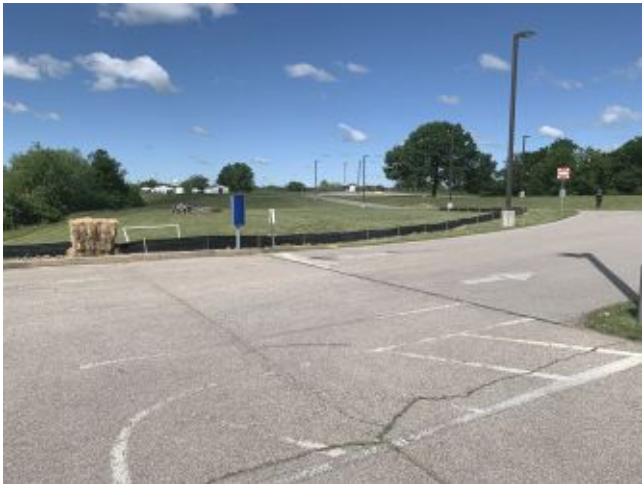
2026.05.04 – Erosion control measures
