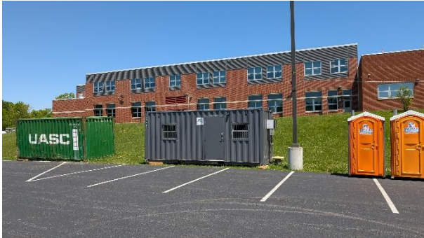
2026.05.12 – Contractor field office, storage, and temporary toilets
