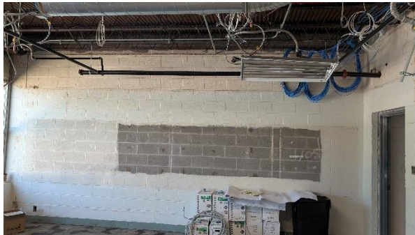
2026.05.12 – Classroom #130 looking east
