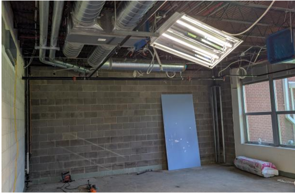
2026.05.12 – Classroom #129 looking east
