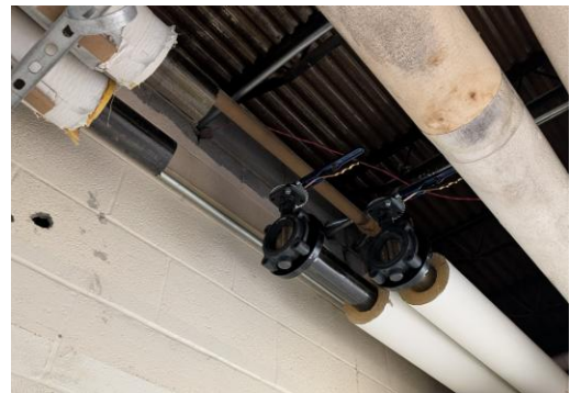
2026.05.12 – Corridor #103 shutoff valve installation
