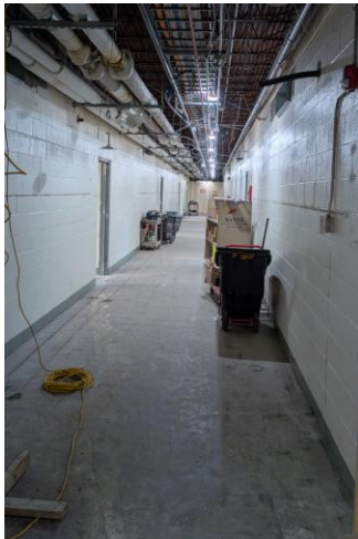
2026.05.12 – Corridor #103 looking west
