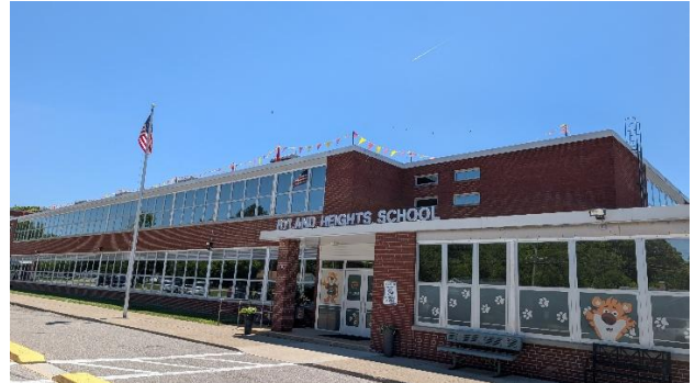
2026.05.12 – Visual Safety perimeter setup on roof
