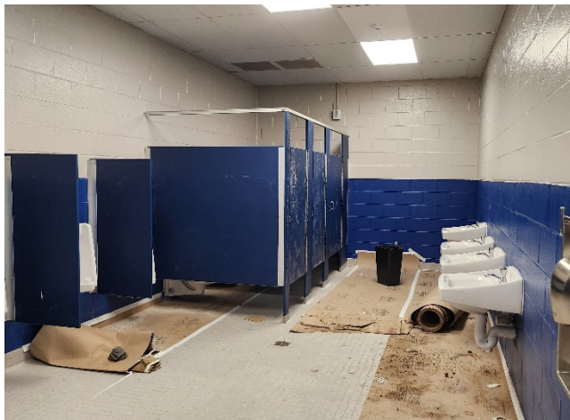
2026.05.06 – Plumbing fixtures and toilet partitions installed in Boys Restroom 156.
