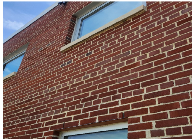
2026.05.06 – Exterior masonry cleaned and sealed. Lintels to be painted.
