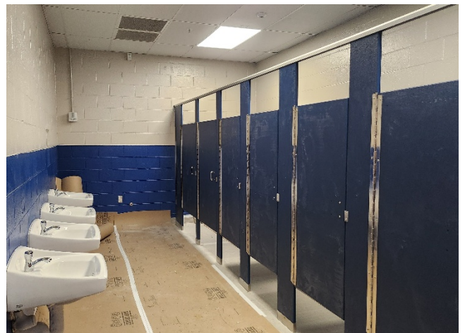
2026.05.06 – Plumbing fixtures and toilet partitions installed in Girls Restroom 155.
