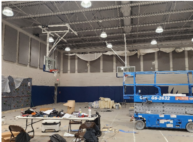
2026.05.06 – Basketball goals, wall pads installed. Walls/ceiling painted. Acoustic panels in progress.
