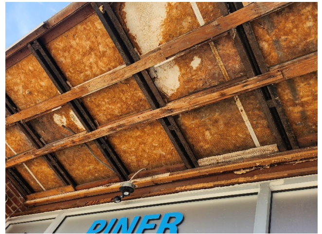
2026.05.06 – Existing soffit panels removed, preparing for installation of new soffit panels.
