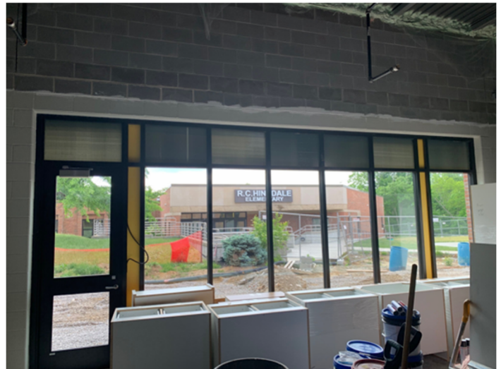
2026.05.05 – New addition – art classroom
