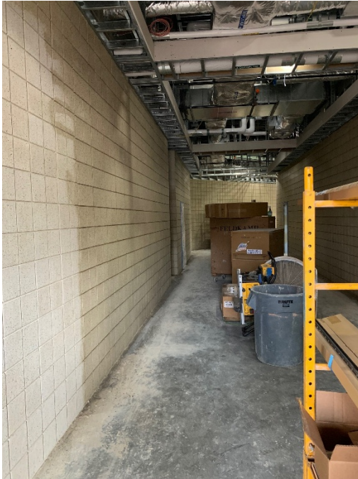
2026.05.05 – Addition main corridor
