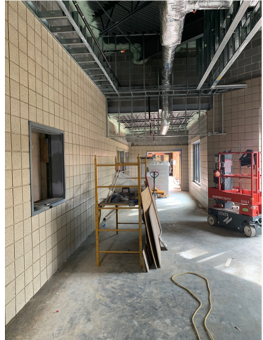
2026.05.05 – Addition main corridor @ ex. bldg
