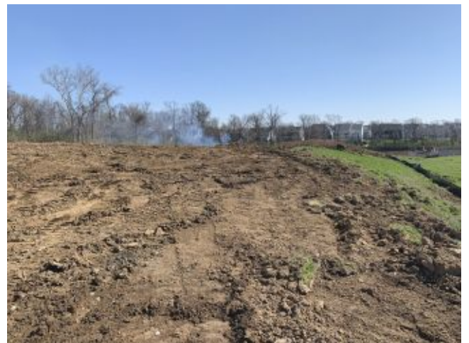
2026.03.24 – Looking east, near existing loading dock
