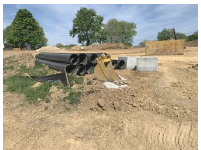
2026.04.21 – Storm piping and structures
