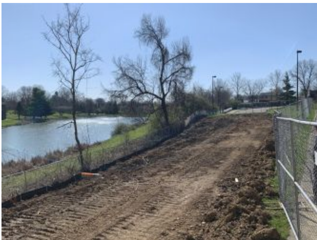
2026.03.24 – Future retaining wall along east side of site
