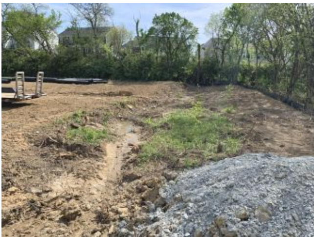
2026.04.21 – South edge of future detention basin
