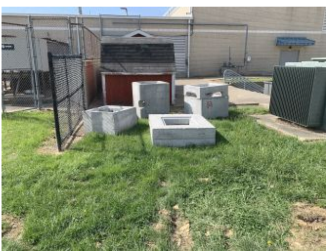
2026.04.21 – Storm structures staged near dock
