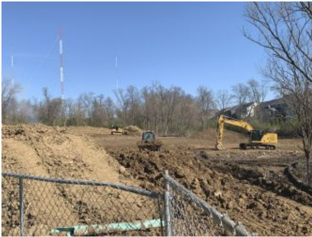
2026.03.24 – Looking north along east side of site
