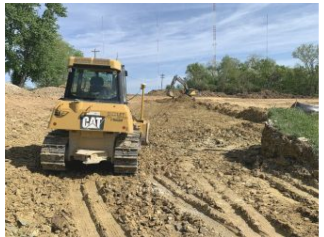
2026.04.21 – Grading at western leg of new drive
