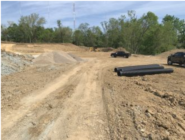
2026.04.21 - Looking north along east side of site
