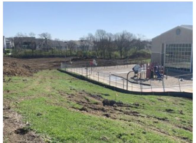
2026.03.24 – Existing playground with temporary fence
