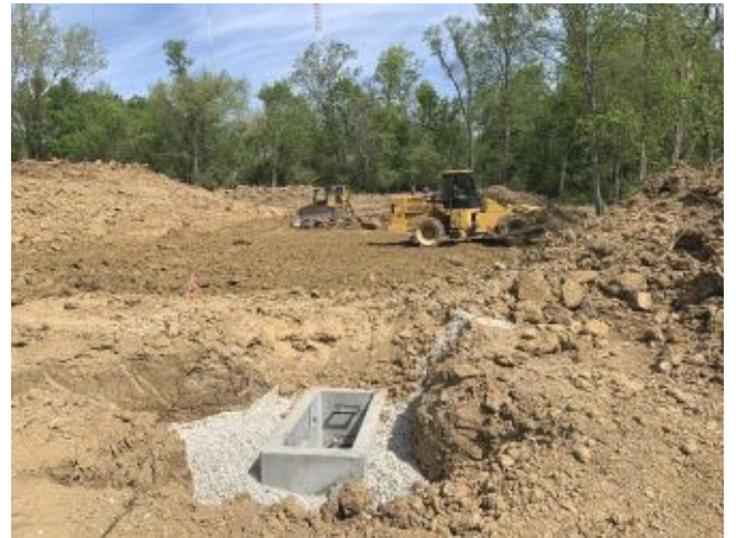
2026.04.21 – Active grading at northeast corner of site
