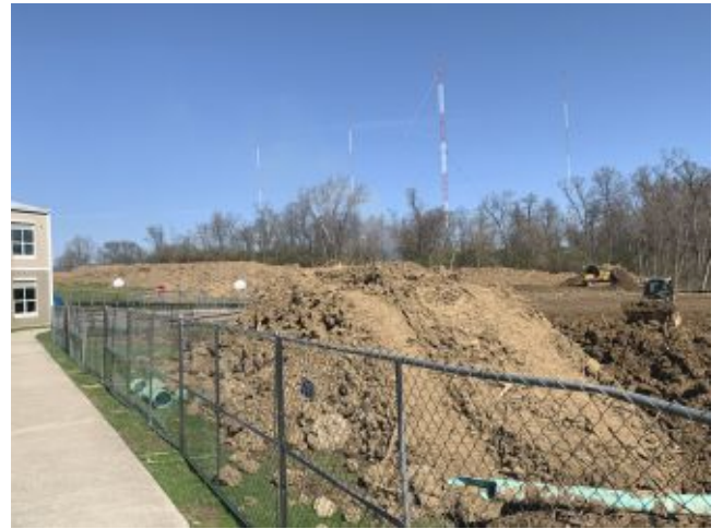
2026.03.24 – Looking northwest from northeast corner of building
