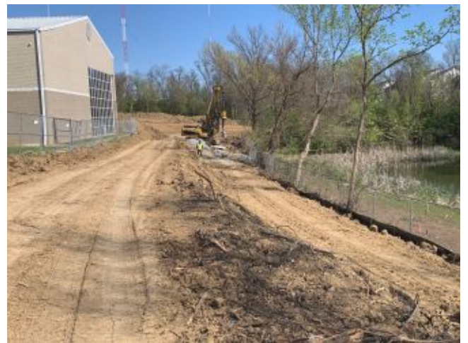
2026.04.07 – Installing drilled piers
