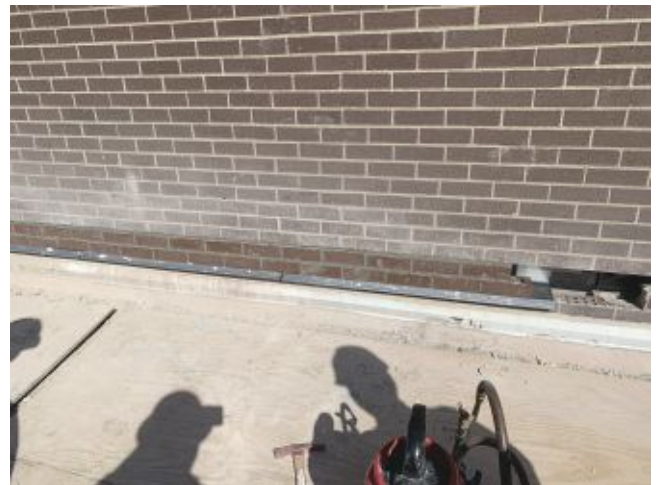
2026.04.16 – Masonry work at Gym
