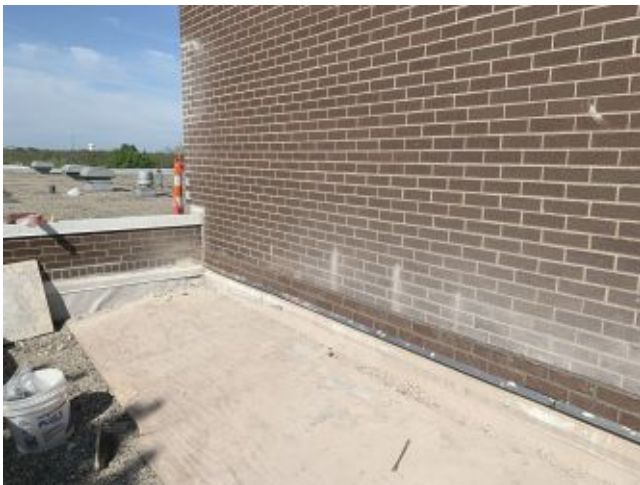
2026.04.16 – Masonry work at Gym
