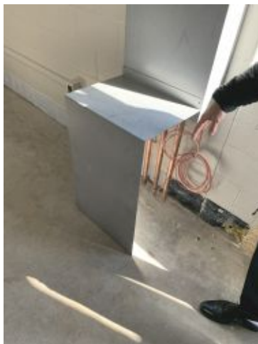
2026.03.19 – Pipe shroud mock-up
