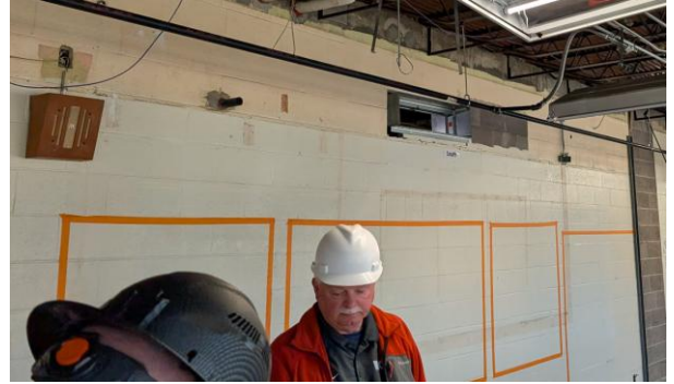
2026.03.30 – Typical Classroom (#126) Mock-up
