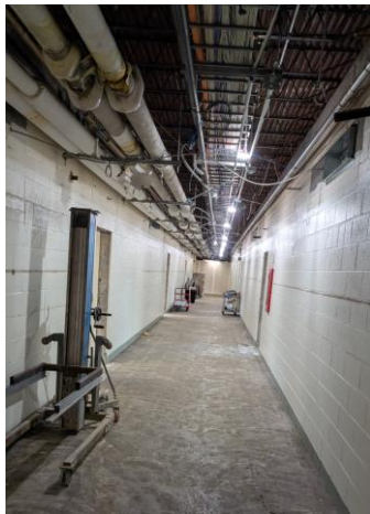
2026.04.14 – Corridor #103 looking west
