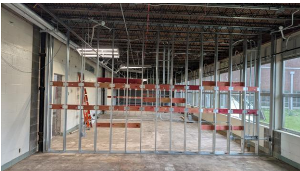
2026.04.14 – Classroom #125 looking east
