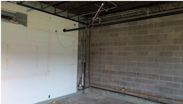
2026.04.14 – Classroom #129 Northeast Corner
