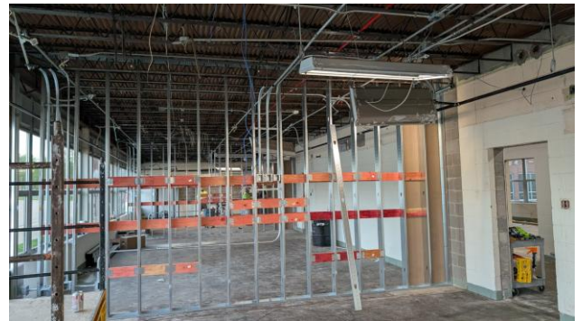
2026.04.14 – Classroom #126 looking east
