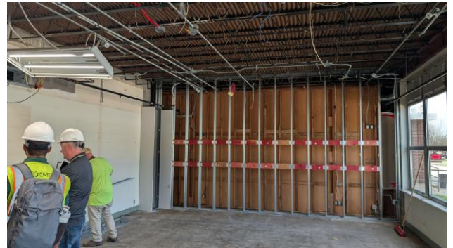
2026.04.14 – Classroom #124 looking west
