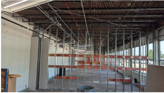
2026.04.14 – Classroom #130 looking west
