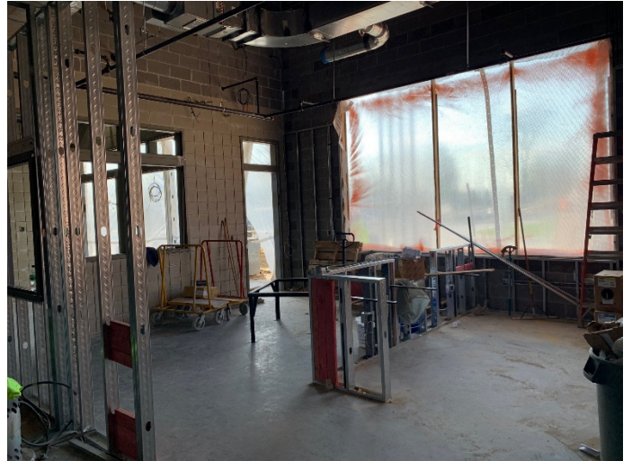
2026.04.07 – New addition reception area
