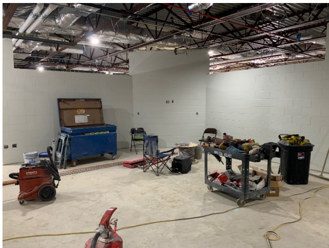
2026.04.07 – Phase 3 typical classroom pod
