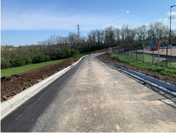
2026.04.07 – Loop road – west side looking north
