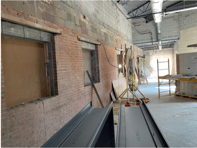
2026.04.07 – New window/door openings to exist corridor
