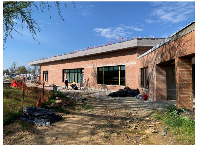
2026.04.07 – New addition – east elevation
