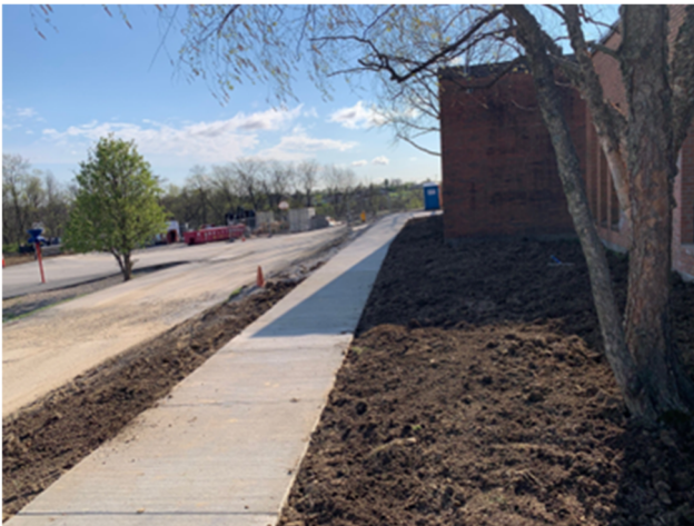
2026.04.17 – New concrete sidewalk from classrooms
