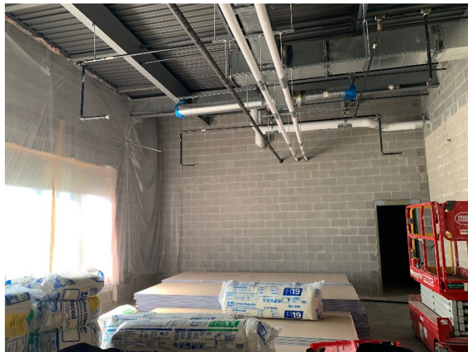
2026.04.07 – New addition – Art classroom
