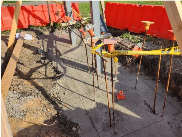
2026.04.14 – Footing and rebar for new marquee sign
