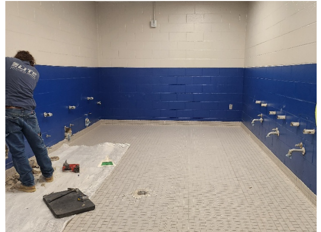
2026.04.14 – Paint and tile in Group C restrooms. Plumbing underway
