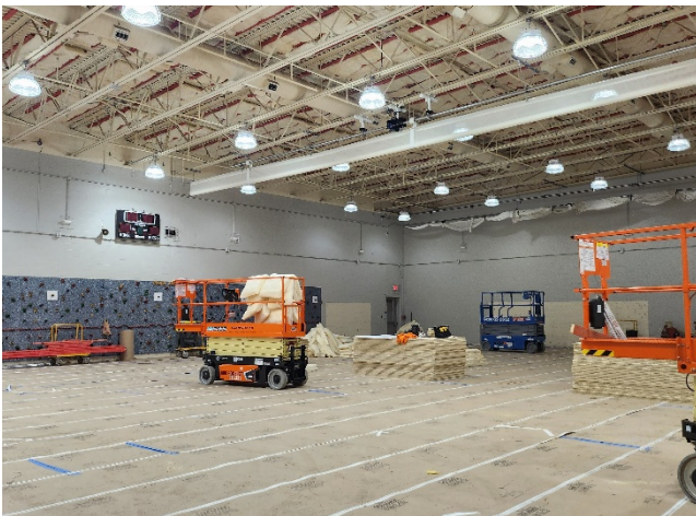
2026.04.14 – Floor protection, new paint in gymnasium
