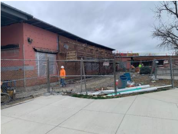
2026.03.10 – New addition exterior-east side
