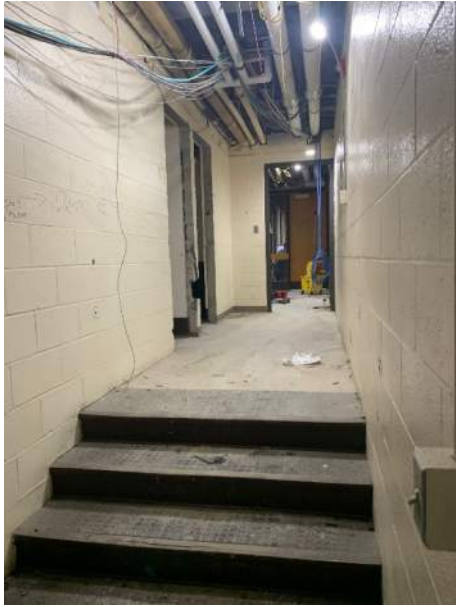
2026.03.10 – Phase 3 corridor demolition
