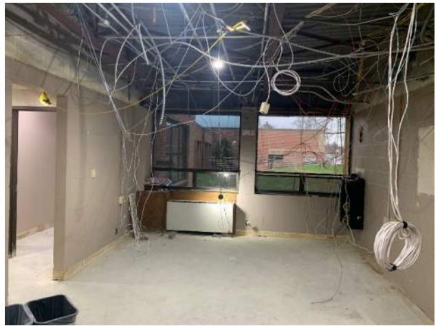
2026.03.10 – Phase 3 office demolition
