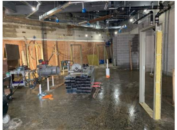
2026.0310 – New addition- main office area
