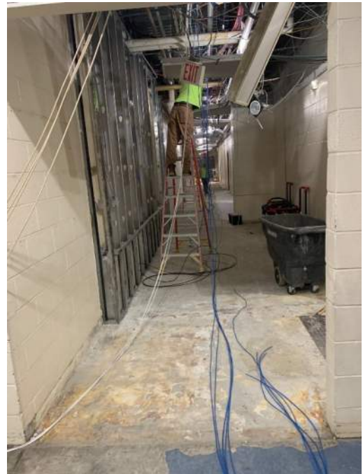
2026.03.10 – Phase 3 Corridor demolition
