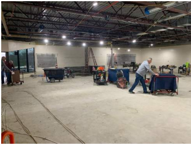
2026.03.10 – Phase 3 Classroom POD demo
