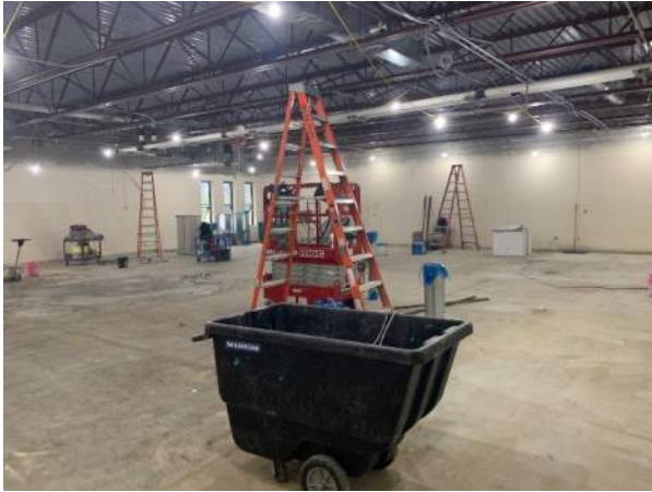
2026.0310 – Phase 3 Classroom POD demolition
