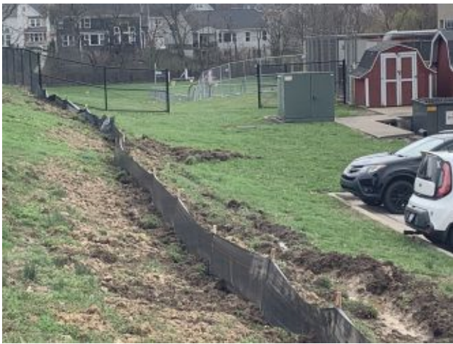
2026.03.10 – Silt fencing. Temporary fence beyond
