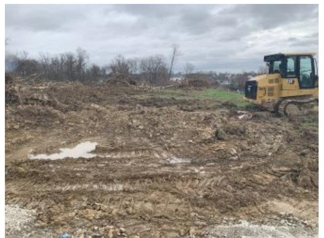
2026.03.10 – Looking east, north of loading dock
