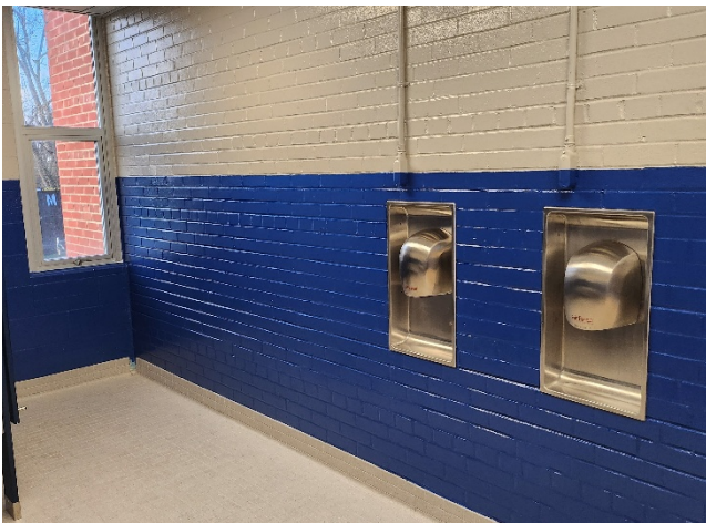
2026.03.12 – New finishes and fixtures in Group B Restrooms
