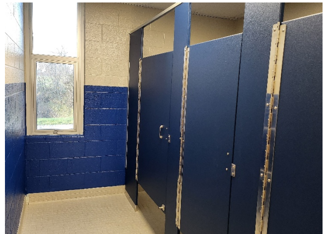
2026.03.12 – New finishes and fixtures in Group B Restrooms
