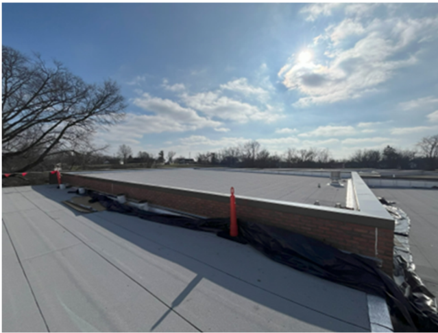
2026.01.13 – New replacement roofing and copings
