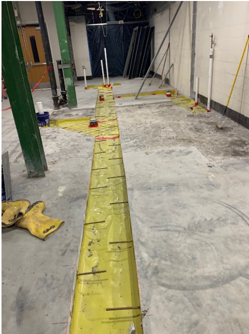
2026.01.13 – Phase 2 Bathrooms underslab rough-in
