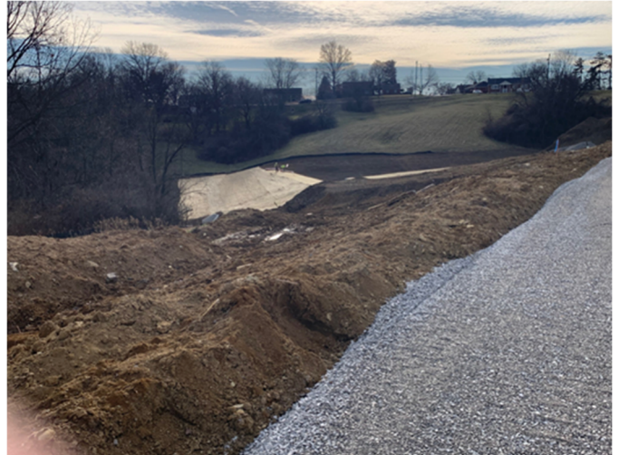
2026.01.13 – Straw mat installation at retention basin
