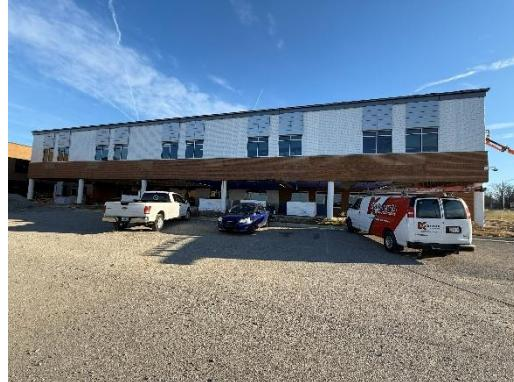
e) The original portion of Area H, which will not be used in the renovation, was mostly removed. This is the north face of Area H which will mate with the south side of the new Area G construction.
