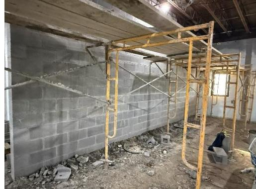
q) The slab at the intersection of Phase 1 on the second floor was too high to meet the existing floor level in Phase 2. Alliance cut down the concrete topping so that the floors in the two phases will be at the same level.
