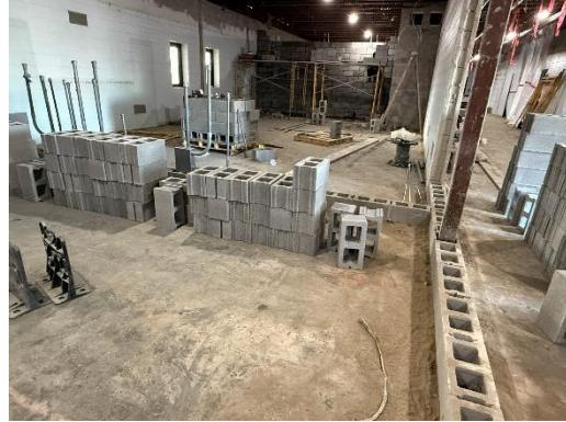
l) The original block walls were laid in stack bond, and where block infill is required the new portions of these walls will also be in stack bond. New walls are laid in running bond. This provides a stronger wall although none of the block walls are structural because of the steel frame in Area H.
