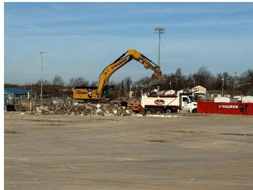
g) Some of the foundation walls were removed so that work can be done on the drive to the loading dock for the kitchen.
