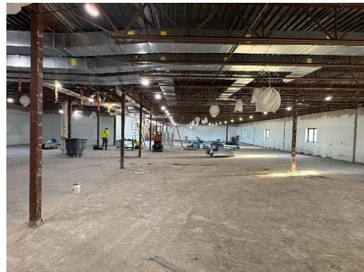
s) Because of the steel structure, the ductwork can be hung without regard for wall openings in walls that were structural in Area J.
