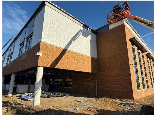
d) The flat composite panels for the parapet were in place on the west side of Area J. The flat composite panels above the windows were also in place.
