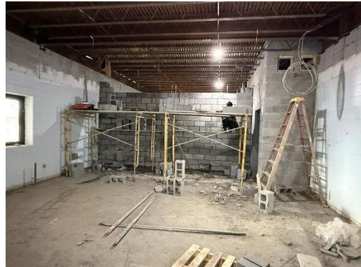
m) New conduits and electrical boxes were being installed in the new walls.
