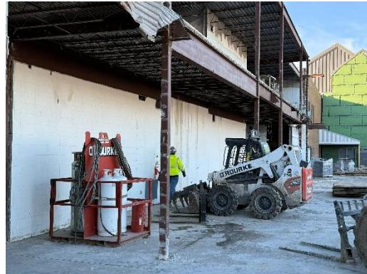
k) New block walls were being laid on the first floor of Area H. The classrooms will be larger to meet KDE standards.
