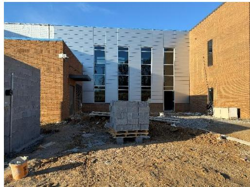
c) Sheet metal workers were installing the flat composite metal panels at the southwest corner of Area J for the parapet.
