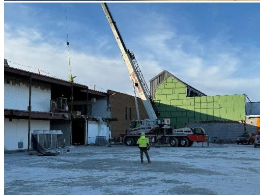
i) Since the original structural framing will be reused, the demolition must be carefully done so that the new structure can interface properly at the original structure.
