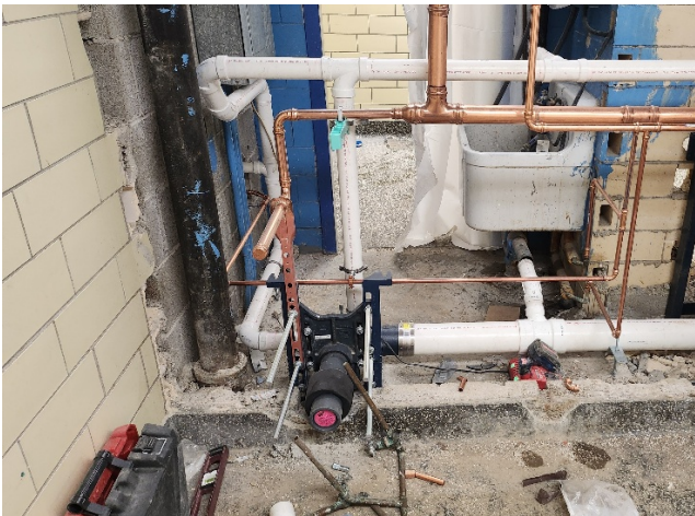
2025.12.09 – New carriers for plumbing fixtures
