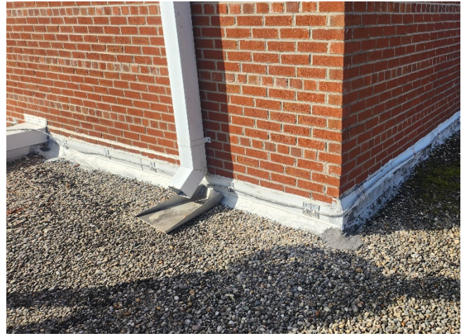
2025.11.04 – Existing weeps covered with caulking
