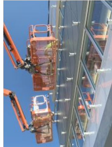
2025.09.30 – Installation of fin rails
