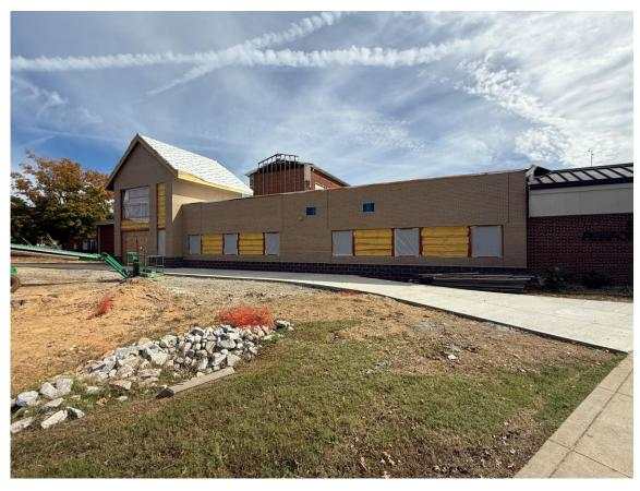
Admin Suite ongoing work includes: Masonry veneer is complete, Electrical and Data installation, wall finishing and paint, floor and wall tiles, ceiling grids and early ceiling tile install, Interior door and window frames.
