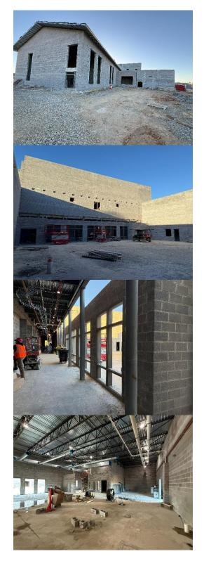
y) The concrete slab had been poured over the precast concrete planks for the north classroom wing. The slabs were protected by the Skudo board system.
