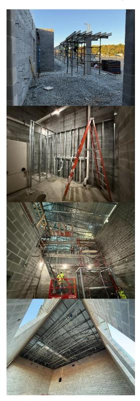
v) Metal angles were installed around openings in the block walls for Area D. This will allow for spray insulation to be applied and then brick.
