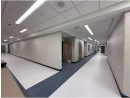
p) The mason had repaired the block walls where the original and new block presented uneven appearance.
