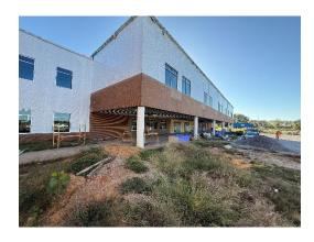
b) Windows in Area J have been installed, and sealant has been applied at all sides.
