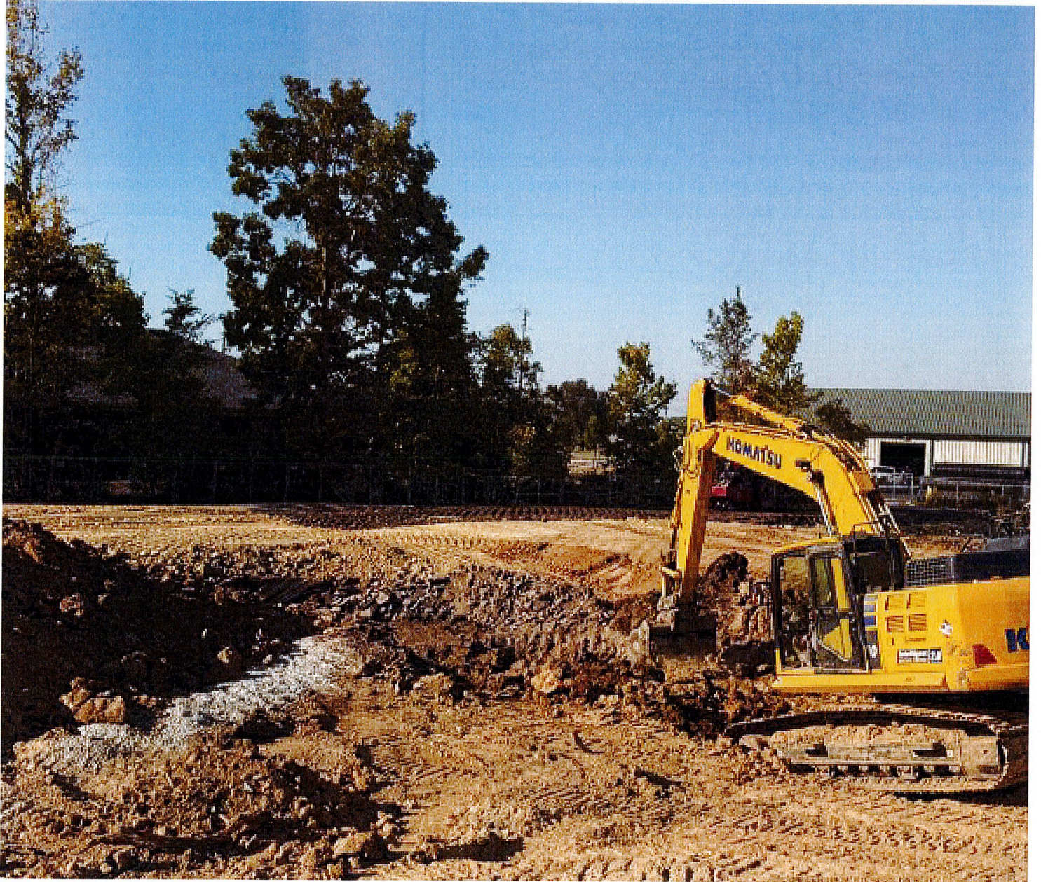
Photo #1: View of undercut excavation.
