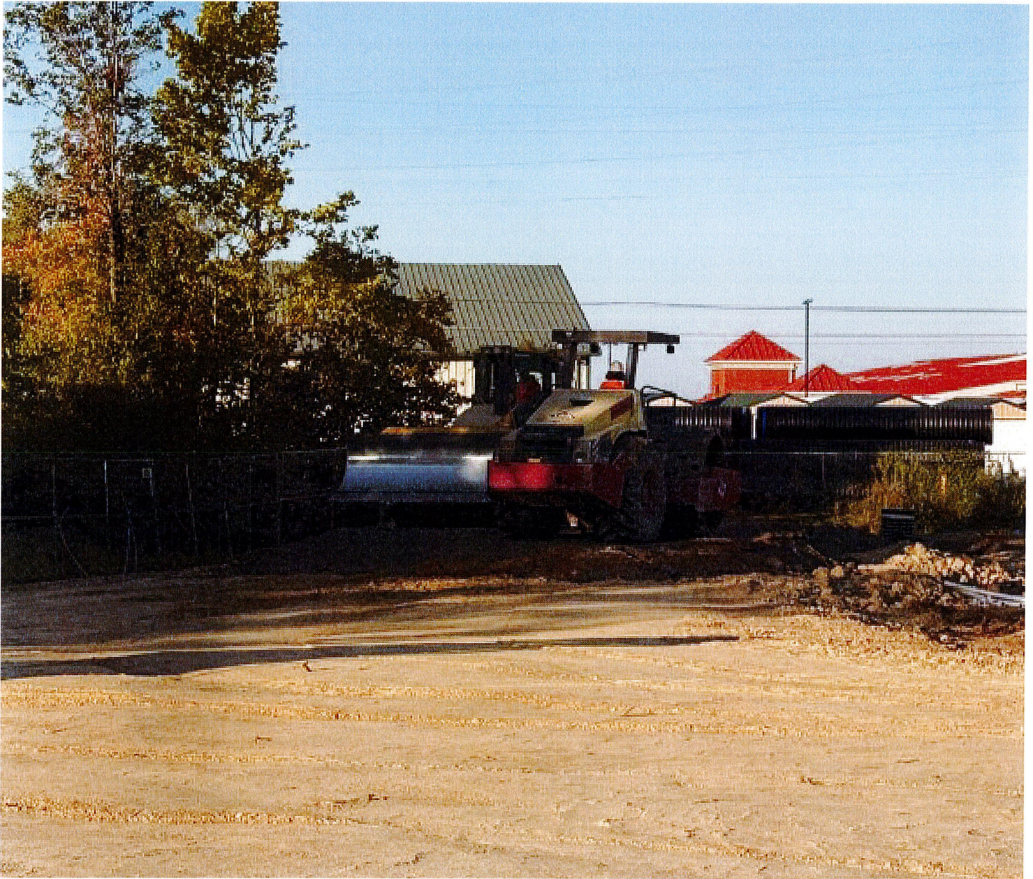
Photo #5: View of fill material compaction.
