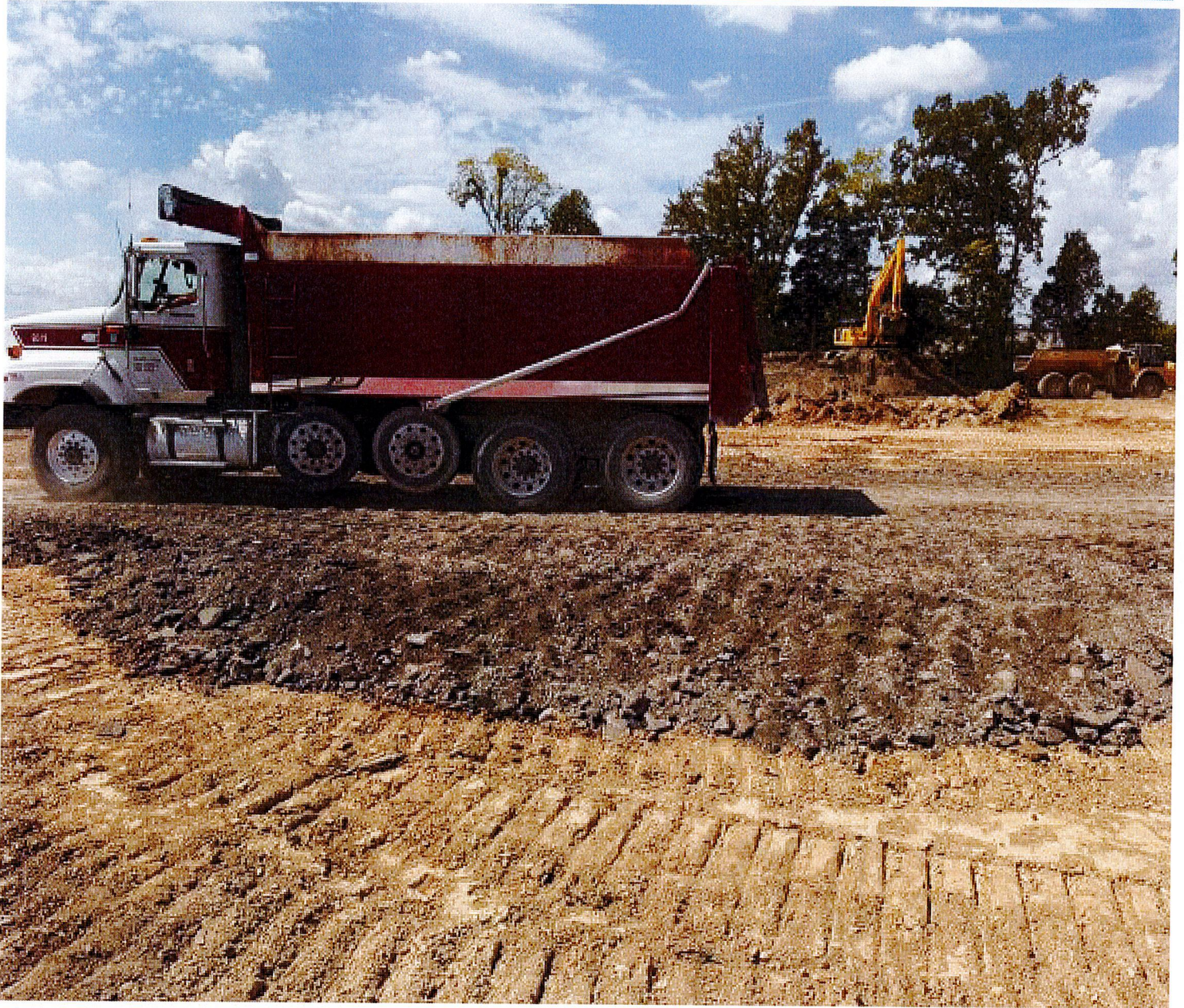
Photo #4: View of truck utilized in subgrade evaluation.
