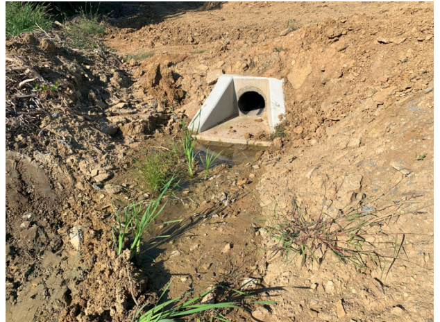
2025.09.09 – New headwall along loop road
