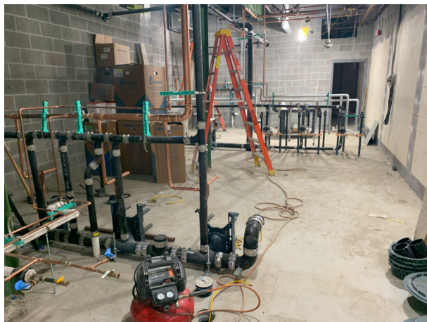
2025.09.09 – Phase 1 area bathroom plumbing rough-in
