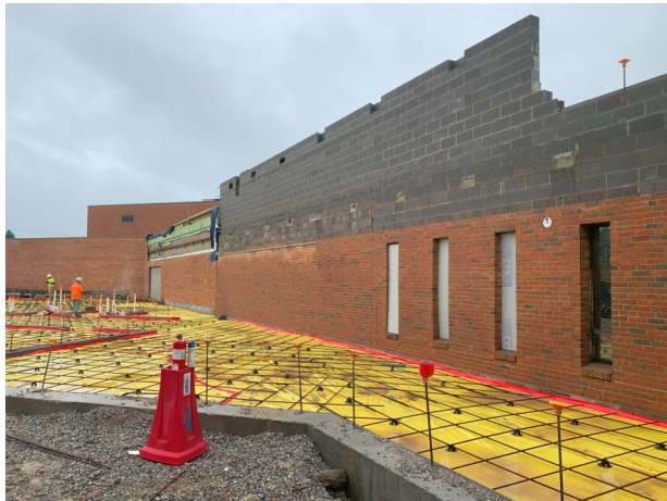
2025.09.23 – New addition slab prep-new cmu wall
