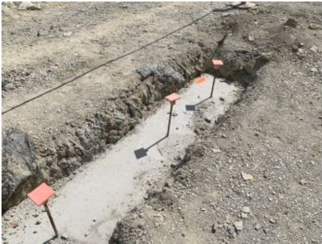
2025.09.02 – Footings for patio benches outside of board room
