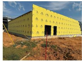
h) Double jamb studs were in place at the hollow metal frames. A single track supported the cripple studs.
