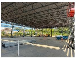
k) The canopy over the loading dock was covered with metal roof deck.
