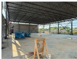
m) Steel channel girts were in place to carry the exterior steel wall panels.
