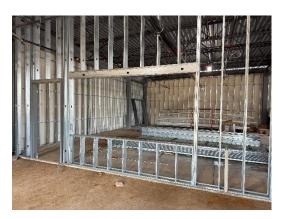
f) Steel bridging was installed in the curtainwall framing at the exterior of the building. The exterior of the framing was being covered with gypsum sheathing panels.
