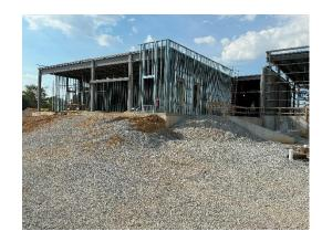
d) Additional light gauge stud framing was in place in the office area. Hollow metal door frames were installed in the wall framing.
