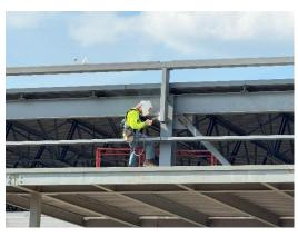
c) Curtainwall framing was installed around most of the office area.
