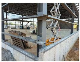
n) Steel framing projected above the roof to form a parapet at the east and north sides of the roof.
