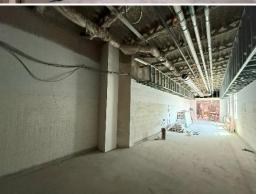
t) The hole in the south stair enclosure above ceiling had not been sealed with block. This is needed for the fire rating for the stair enclosure.
