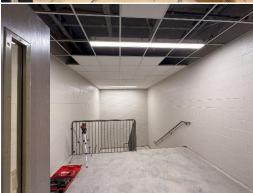
s) The wall where the original lockers were removed was repaired.
