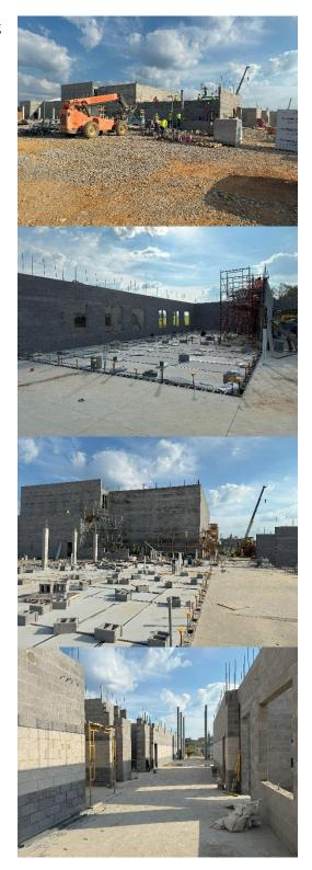
k) The ground faced concrete blocks stop at the top of the metal door frames. The walls will be painted above that. The outside corners have a bullnose radius.
