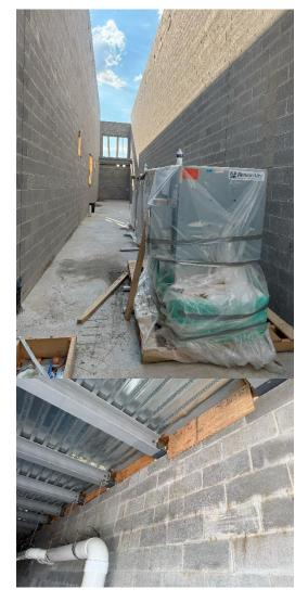
z) Fire treated plywood was used to close the ends of the rood deck for the slab pour. This needs to be reviewed with the building inspector. This is only visible above the mechanical platform.
