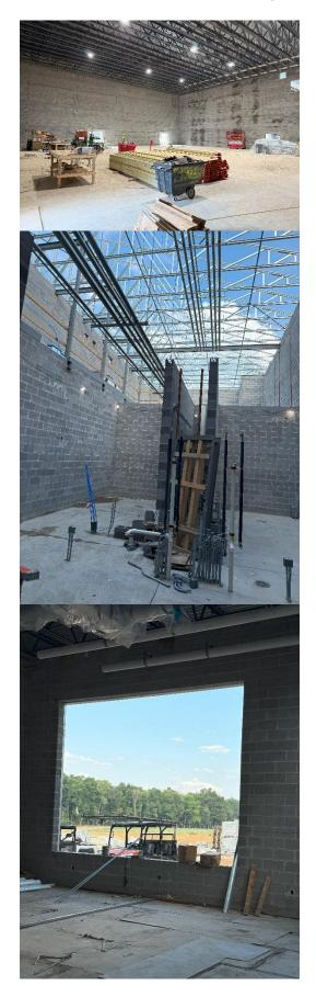
u) Corrections to this opening and another at the Area D corridor were underway. Steel reinforcing. Jamb blocks and the lintel need to be installed according to the structural drawings. When repaired, the walls must match the surrounding block spacing and texture.
