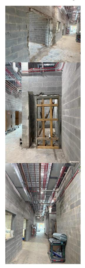
v) Piping and ductwork for the Area D corridor were installed. This area is in the storm shelter. All penetrations that run through storm shelter walls must meet the specific requirements and details for each penetration.
