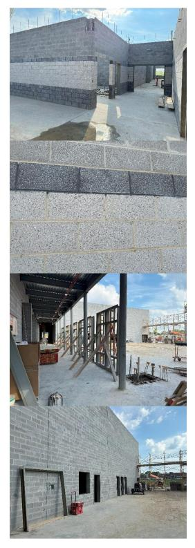
r) The gym roof area is now covered with the concrete slab. This will effectively dry in the space, although the roofing system will need to be in place to completely keep water out.
