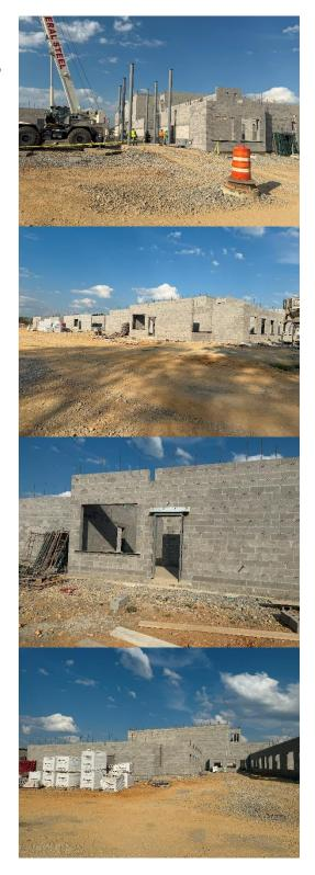
g) The southernmost classroom wing was being laid up with concrete block.
