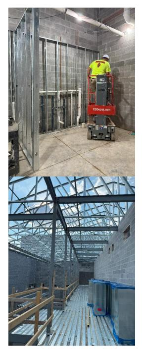
y) The concrete slab for the mechanical platform on the north side of the gym was in place. HVAC units were being stored near where they will be installed.
