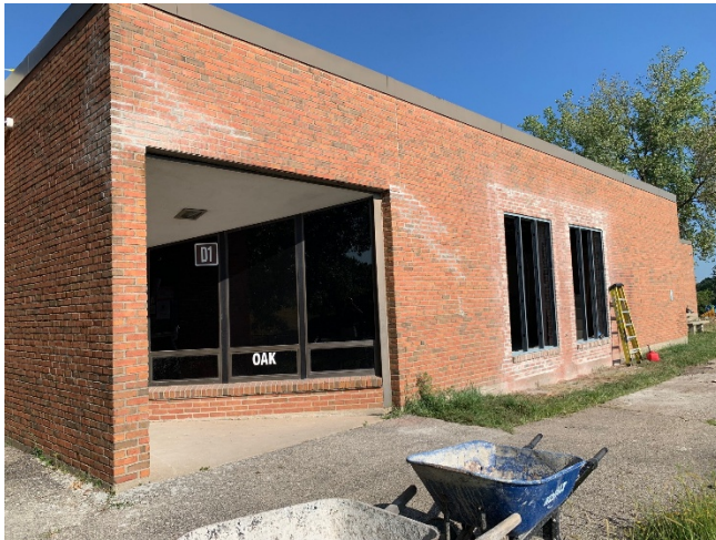
2025.87.13 – Brick tuckpointing/repair
