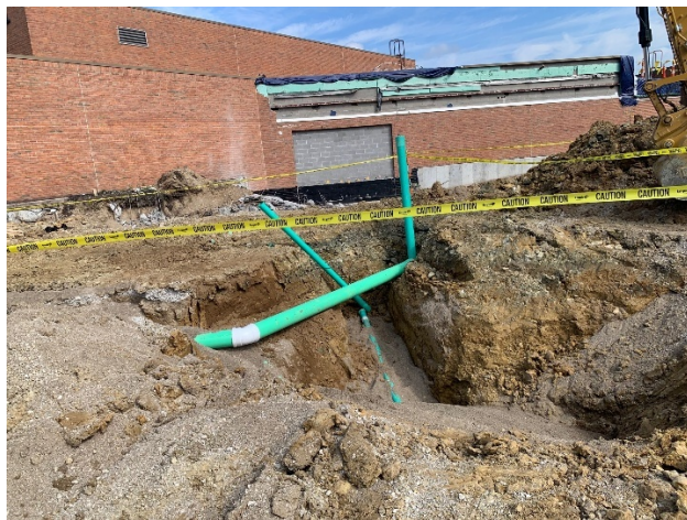
2025.07.15 – Storm piping installation at new addition
