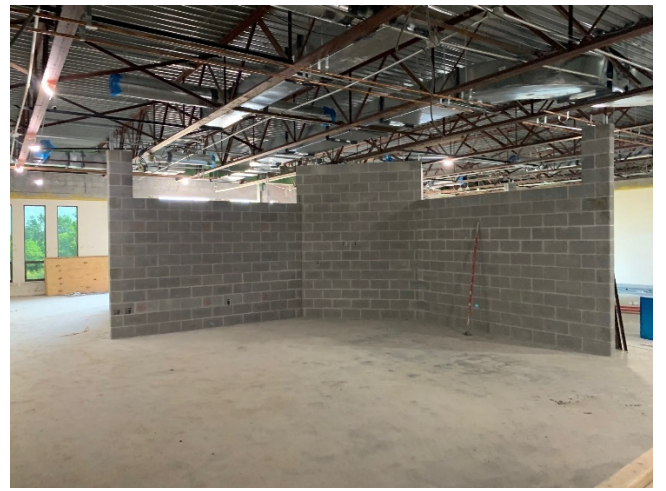
2025.07.29 – New cmu walls – typical phase 1 classroom pod
