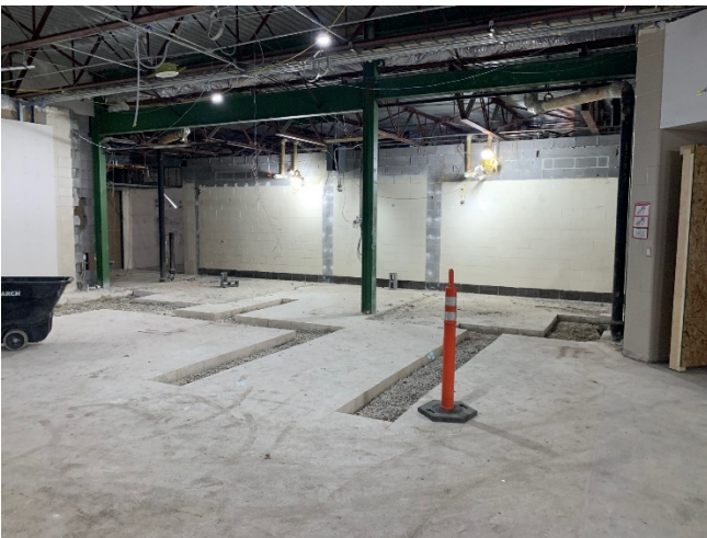
2025.07.29 – Slab removal for bathroom plumbing-phase 1
