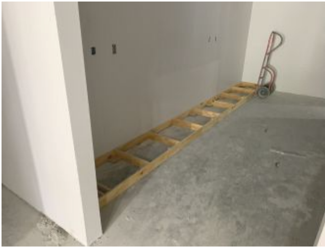
2025.08.05 – Casework toe kick framing in Work #122
