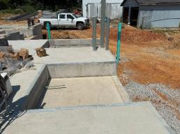
g) The pit for the dock leveler into the warehouse appeared to be ready for the leveler. A conduit was extended into the pit for the leveler motor.
