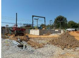
d) The concrete crew was preparing the area for the transformer and generator.
