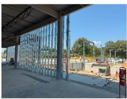
j) The corridor in front of the freezer was bordered with the pressure treated wood blocking that will be under the front wall of the freezer.
