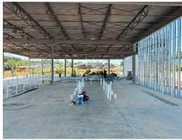
i) Light gauge structural exterior wall framing was extended past the east wall of the warehouse.
