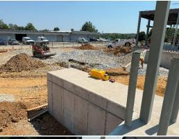
f) The pit for the dock leveler on the loading dock appeared to be ready for the leveler. A conduit was extended into the pit for the leveler motor.
