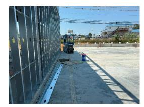
l) Steel columns were being installed in slab block outs in the warehouse area.
