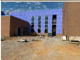
d) Two different colors of air barrier were in place due to availability of the original material.
