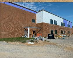
e) The air barrier was being completed on the south elevation.
