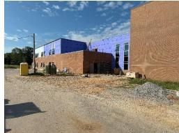
c) The connector to Area H was being prepared for the sheet metal panels. The curtainwall windows were mostly installed.
