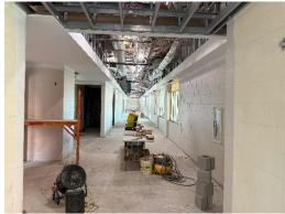
j) Soffit framing was being installed in the connector to Area H.
