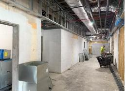
r) Repair work is required at the duct openings in the load bearing block wall between the steel beam and floor above.
