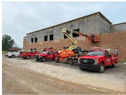
o) The brick was being replaced where the flashing for the canopy over the exit doors was removed.
