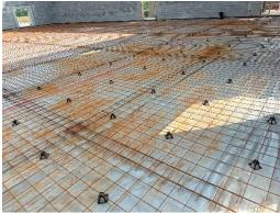
Defore the concrete is poured the vapor barrier is required to be taped to the block walls. This reduces moisture rising into the wood gym flooring system.
