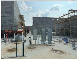
o) It appeared that the insulated concrete slab was poured to form the base for the walk-in cooler and freezer off the Kitchen.
