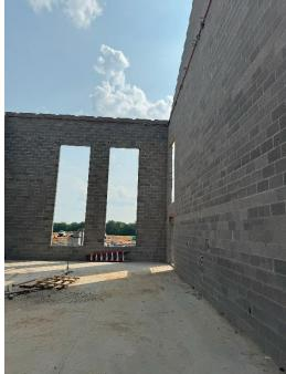
g) Interior walls for rooms off the Band Room, including the practice rooms and office were laid, and the door and window frames were installed.
