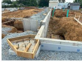
i) Due to the depth of the footings at the loading dock wall, a considerable amount of fill is required.
