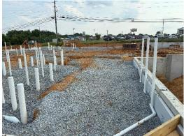
g) Leave outs for steel column base plates were formed. The loading dock foundation wall was poured and the forms removed.
