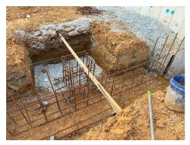
Forms were in place for the retaining walls at the maintenance building loading dock.
