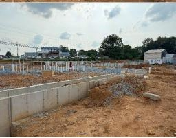
f) Rigid perimeter insulation was installed against the foundation walls and the area back filled with crushed stone.
