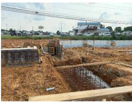
k) Steel reinforcement was in place for the foundation supporting the columns in the warehouse.
