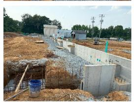
j) The foundation between the office area and the warehouse was being prepared with the steel reinforcing being placed. Construction of this foundation was delayed until the rest of the under-slab work was in place to allow construction equipment access to the office area.
