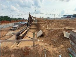
c) Forms had been removed from the foundation walls around the office area.
